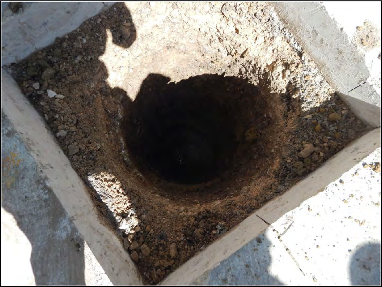
Figure 4-4. Borehole for bus shelter pier along the San Pedro Creek.
