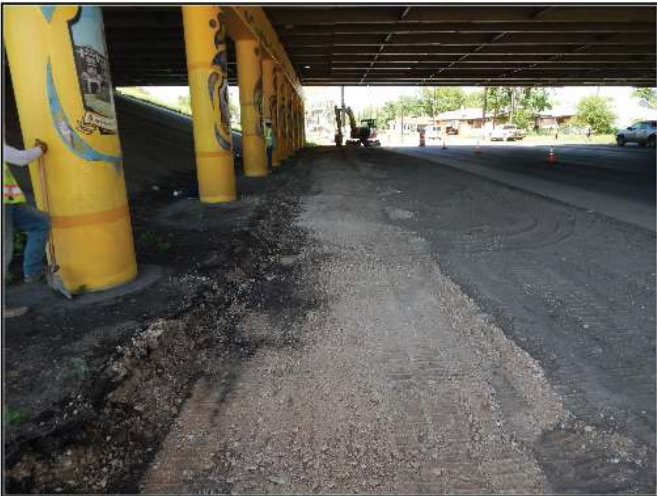
Figure 4-2. Excavation at Roosevelt Avenue underpass.
