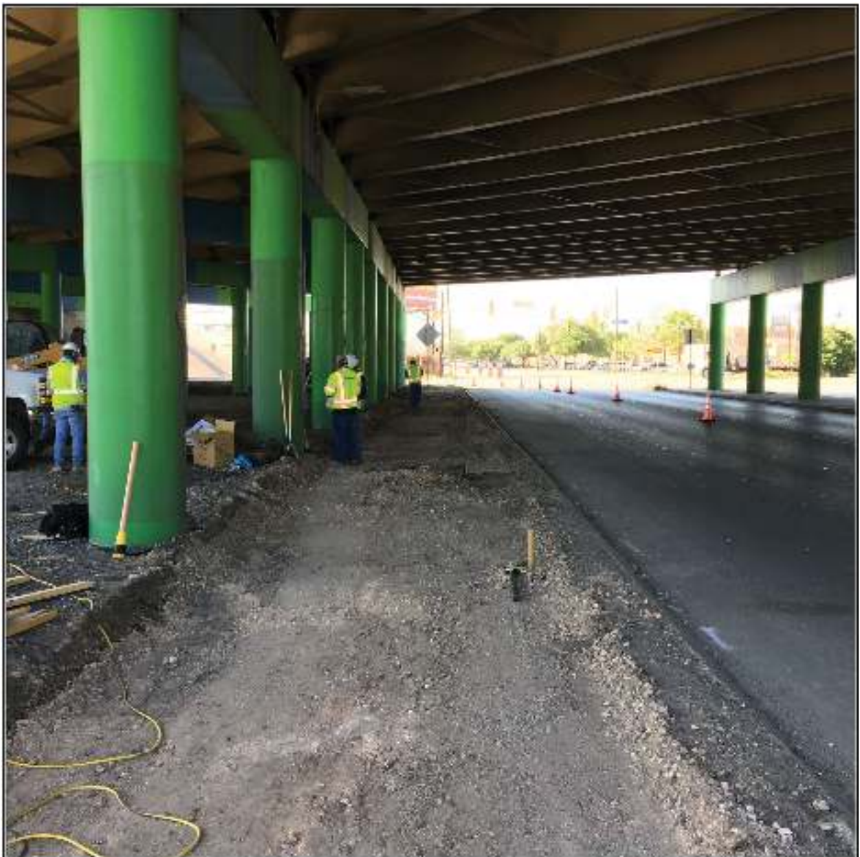
Figure 4-1. Sidewalk excavations at Mission Road and Steves Avenue.
