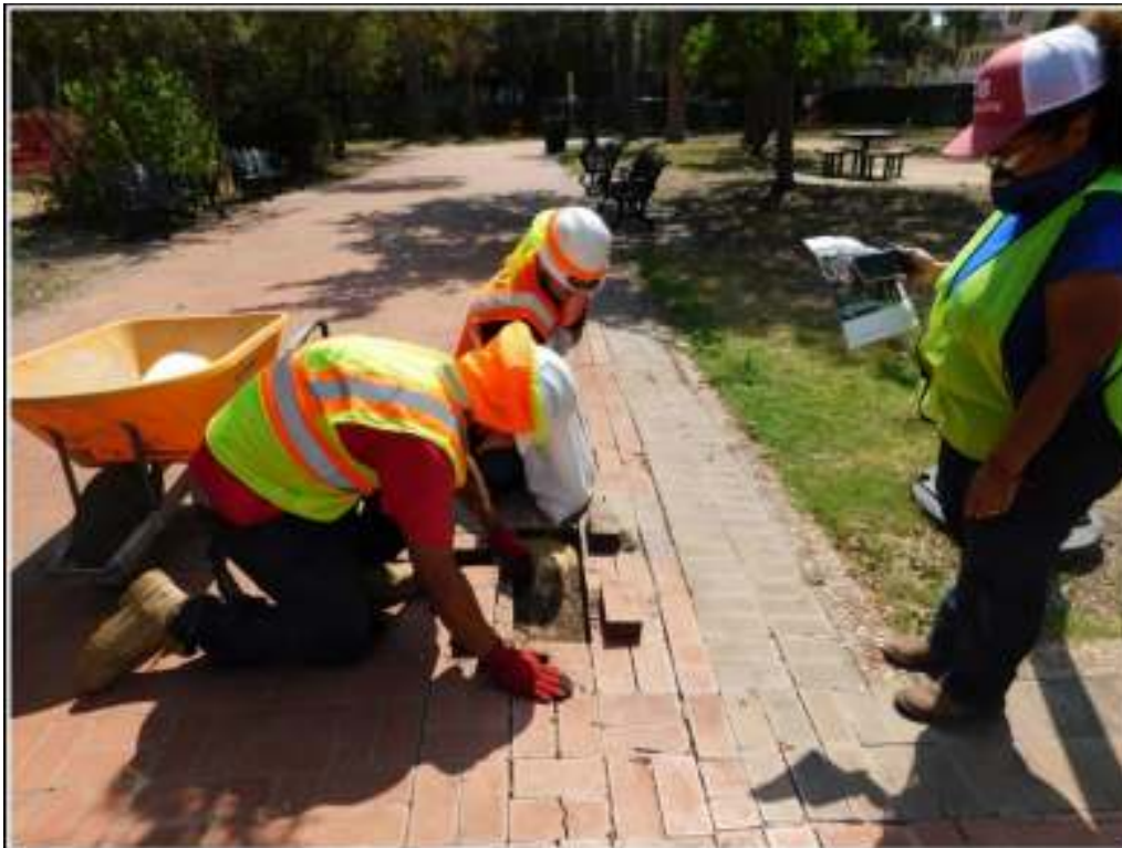
Figure 3-3. Paver repair near the gazebo and playground.
