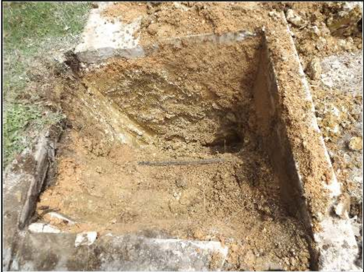
Figure 4-6. Excavation within Project Area 4 on Euclid St.
