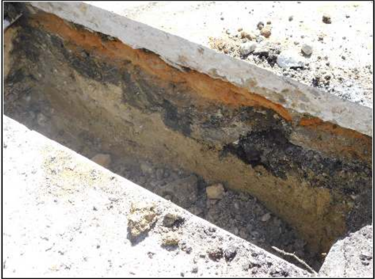
Figure 4-4. Pit excavation within Project Area 2 near Flores Street and Park Court.
