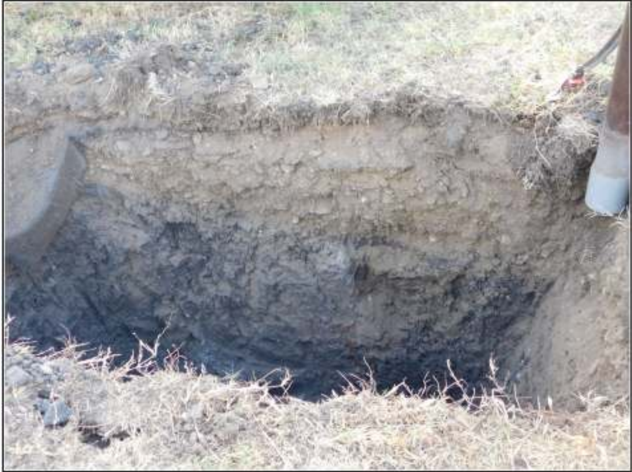
Figure 4-10. Excavation within Project Area 7 on Martin Street.
