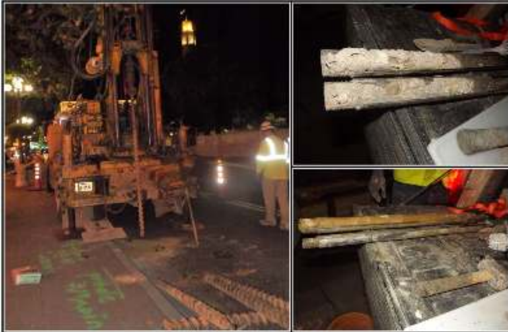
Figure 4-2. Boring of B-1 in progress; sample 1 (top right) and sample 7 (bottom right).
