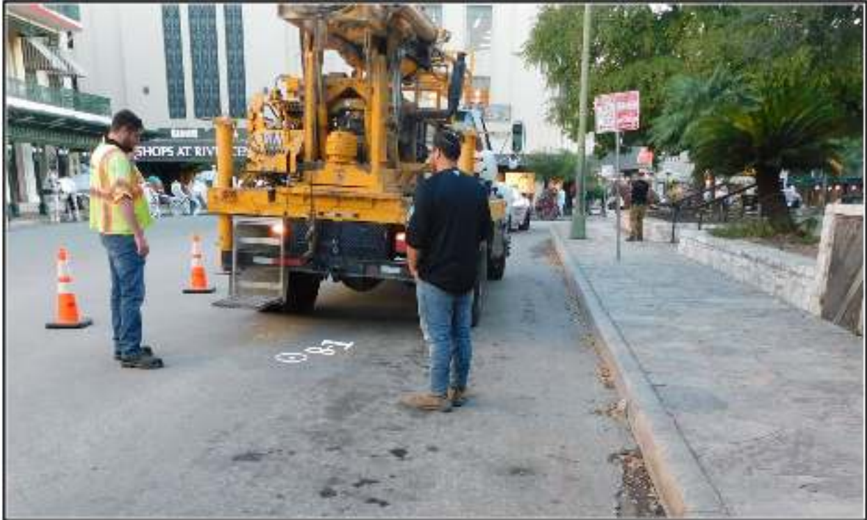
Figure 4-2. Terracon and Ramco crew setting up for B-1.
