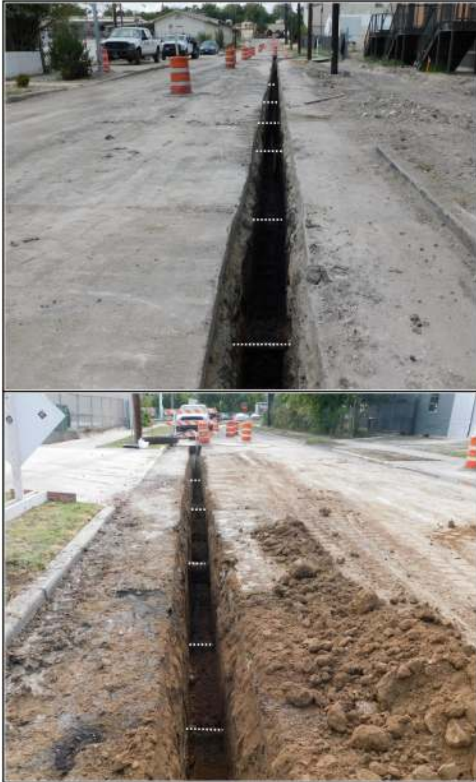
Figure 4-2. Trenching along west and east ends of the APE. Numerous utilities cross the trench and are highlighted by dashed lines (white).
