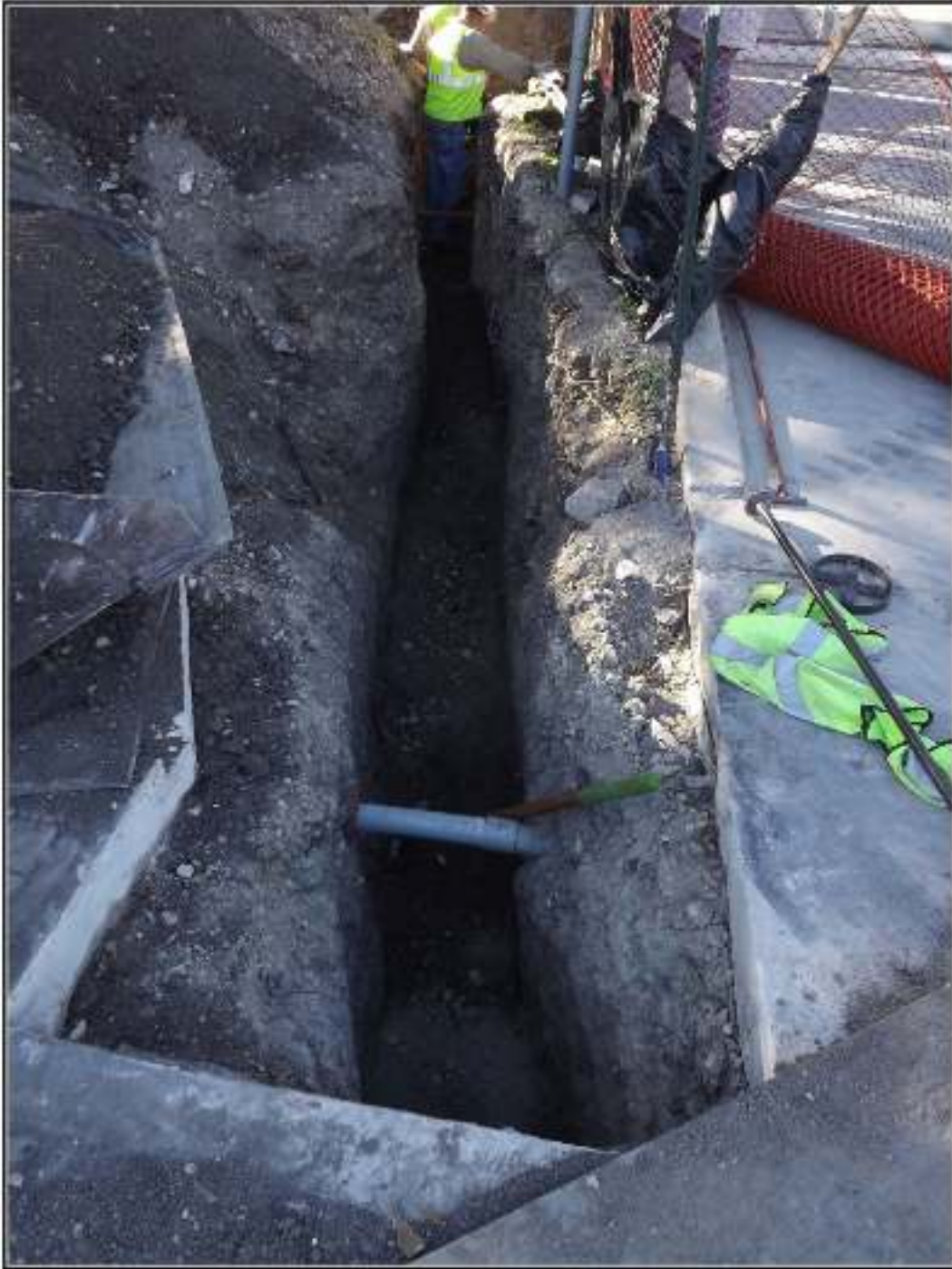
Figure 3-3. Southeastern portion of Trench Section 2 ending at edge of the sidewalk.
