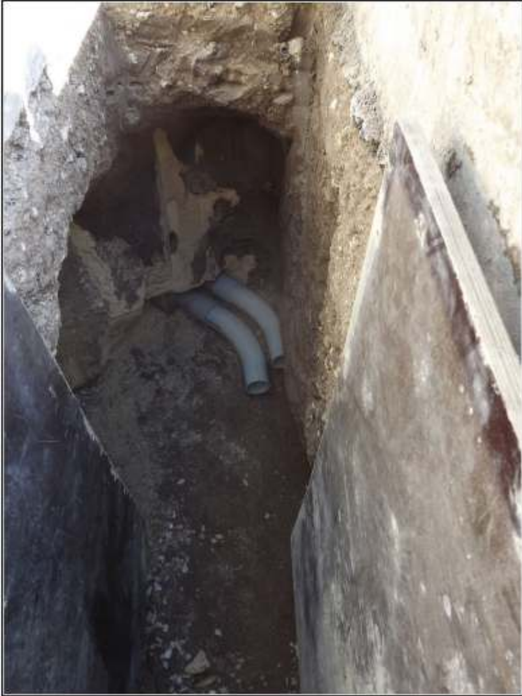
Figure 3-5. Southeastern portion of Trench Section 3 connecting to manhole structure.
