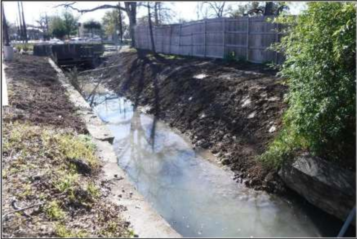
Figure 4-7. The canal banks after the application of topsoil (facing southeast).
