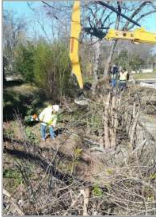
Figure 4-2. COSA crew manually and mechanically removing vegetation from the canal.
