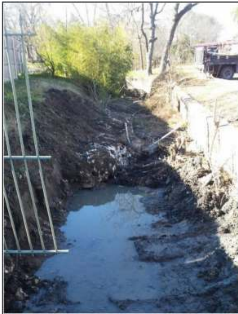
Figure 4-6. The canal after Stage 1 (facing west).
