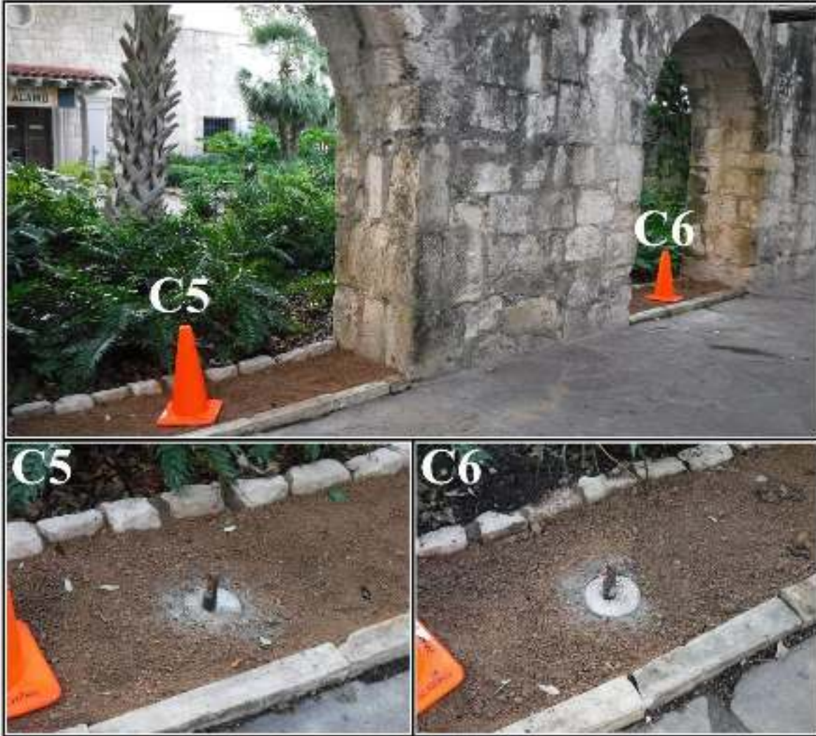
Figure 4-4. C5 and C6 locations prepared for cannon installation (facing south).
