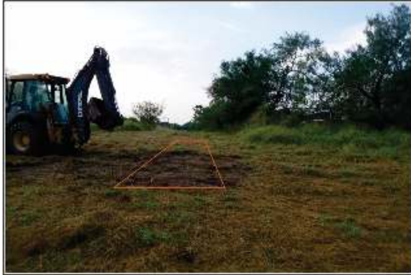
Figure 4-7. BHT 3, prior to excavation. Location outlined in orange.
