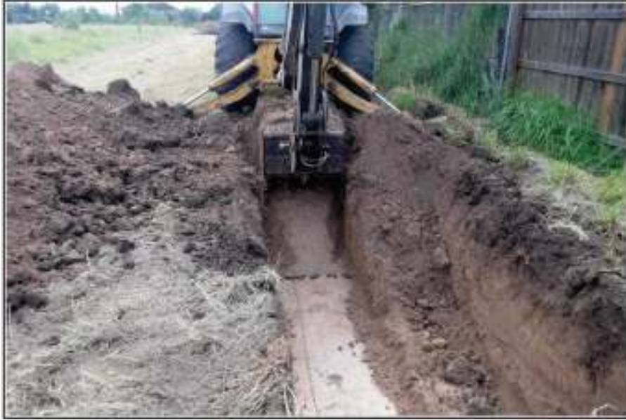
Figure 4-4. BHT 2, excavation in-progress.
