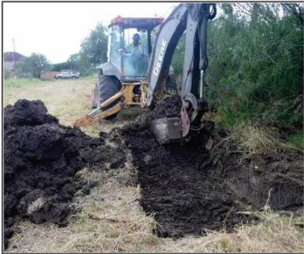
Figure 4-2. BHT 1, excavation in-progress.
