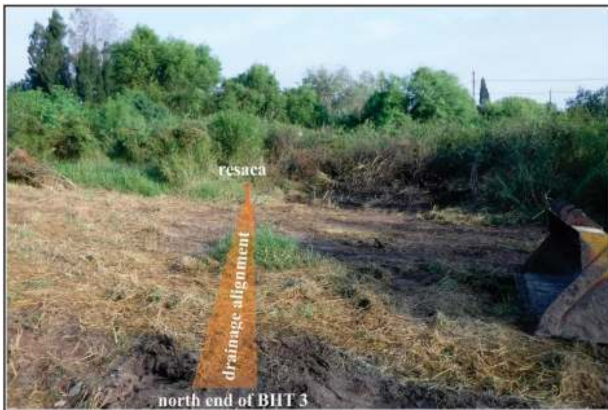
Figure 4-6. North end of proposed drainage alignment at the resaca.
