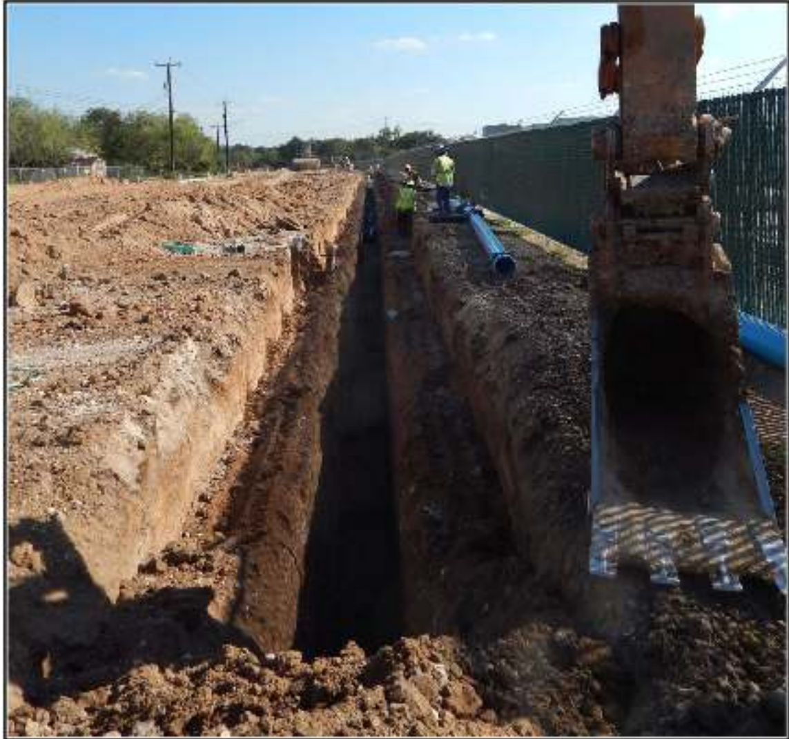
Figure 4-2. Area 1 viewed south from Rilling Road.
