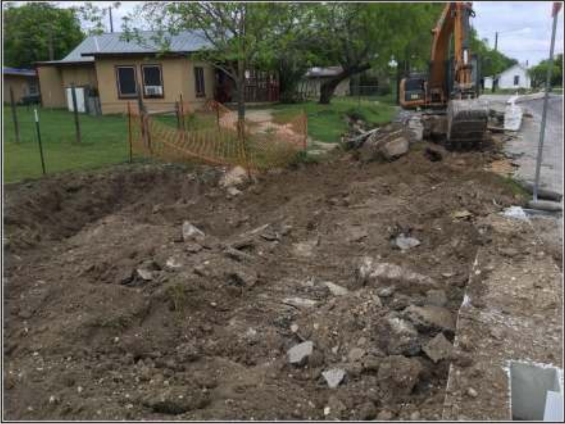
Figure 4-5. View to the northwest of excavation for waterline in Area 2.
