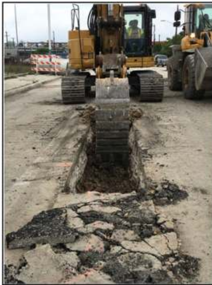
Figure 4-2. Excavation of main SAWS utility prior to blacktop removal (facing south).
