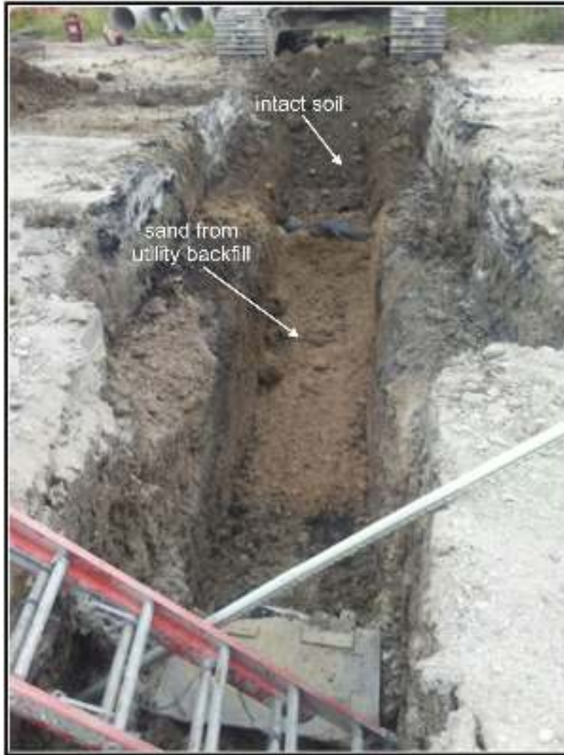
Figure 4-4. SAWS lateral excavations, note differences in soils.
