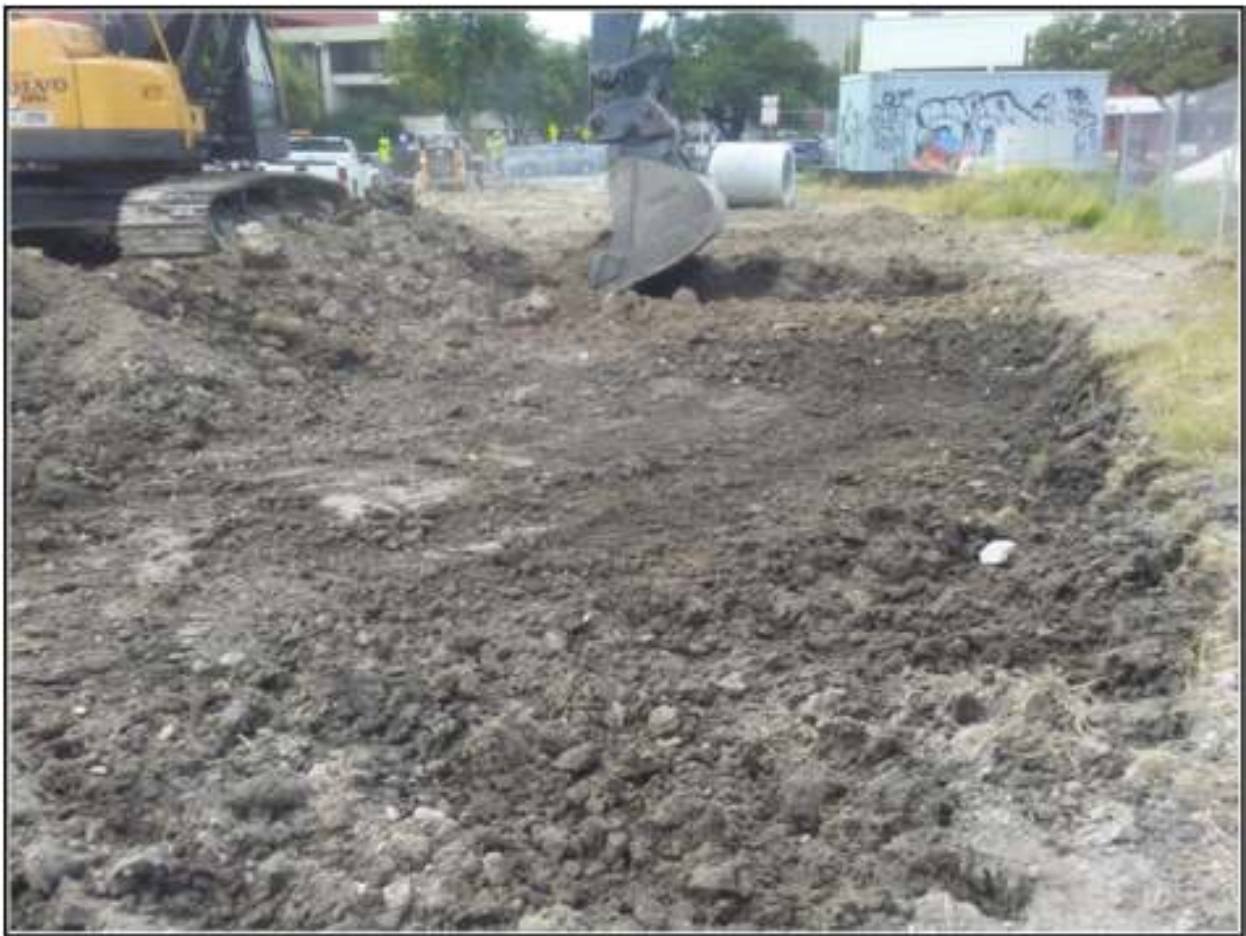
Figure 4-5. COSA road grading with large excavator (facing south).
