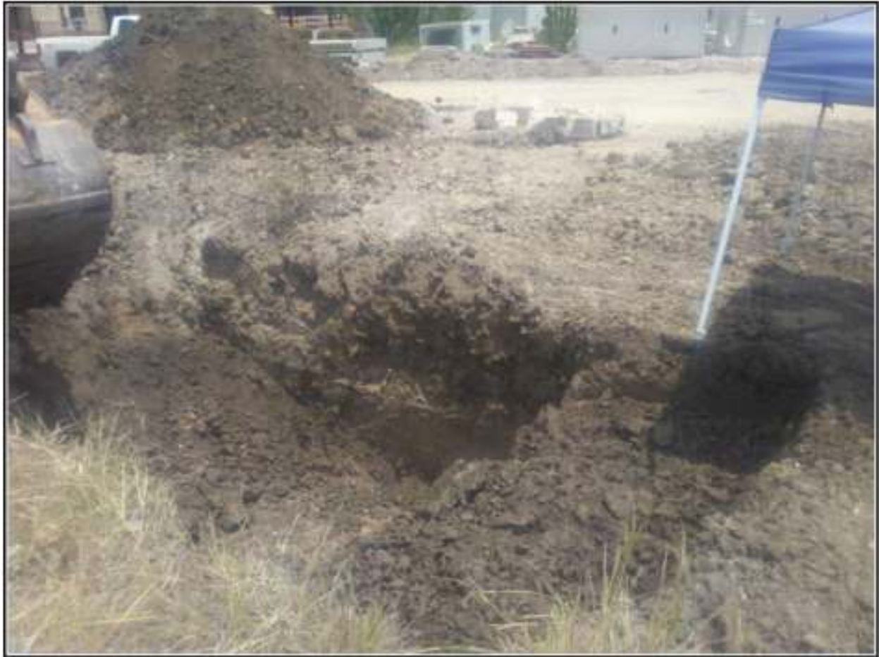
Figure 4-6. Storm sewer excavations for COSA.
