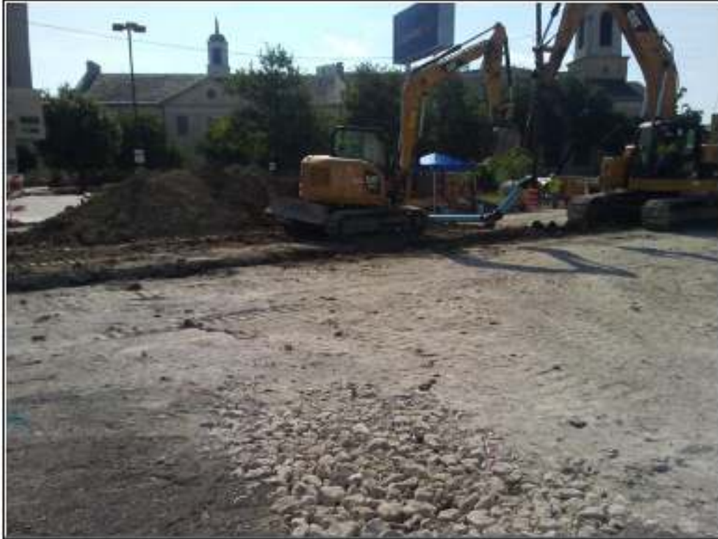
Figure 4-3. Photograph of main SAWS water utility trench and installation of pipe.
