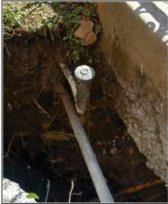
Figure 4-6. Utilities in Trench 3 where cultural material was observed.
