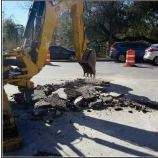
Figure 4-2. Trench 1 excavated for CPS Energy line, connecting to manhole.
