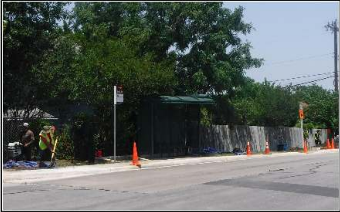
Figure 4-3. Hand-excavated trenches along the north side of Yucca Street (view northeast).
