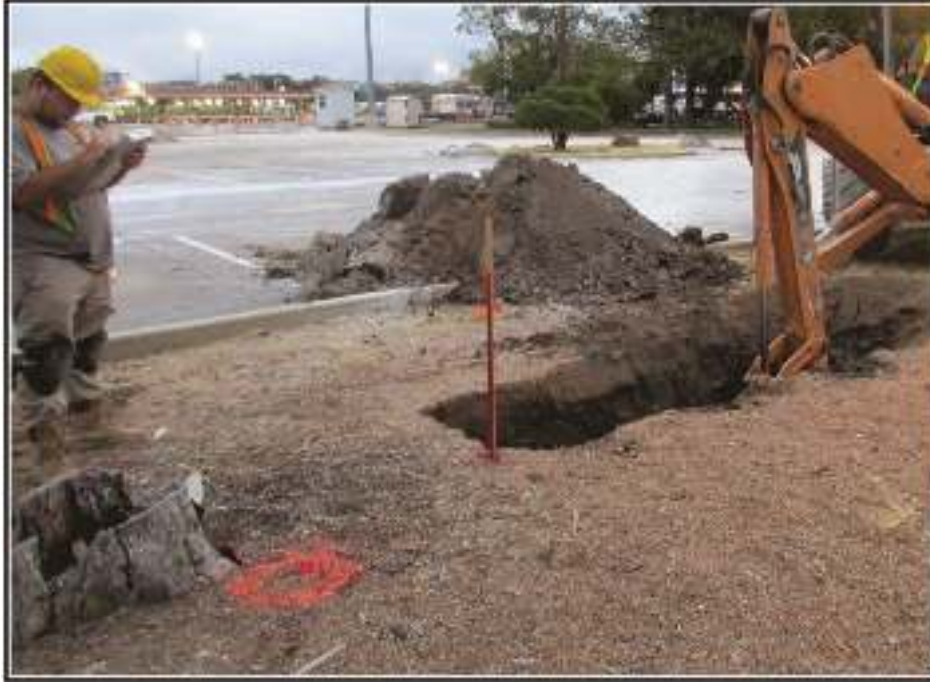
Figure 4-6. BHT 3, trenching in progress, facing northeast (Nov. 1, 2016).
