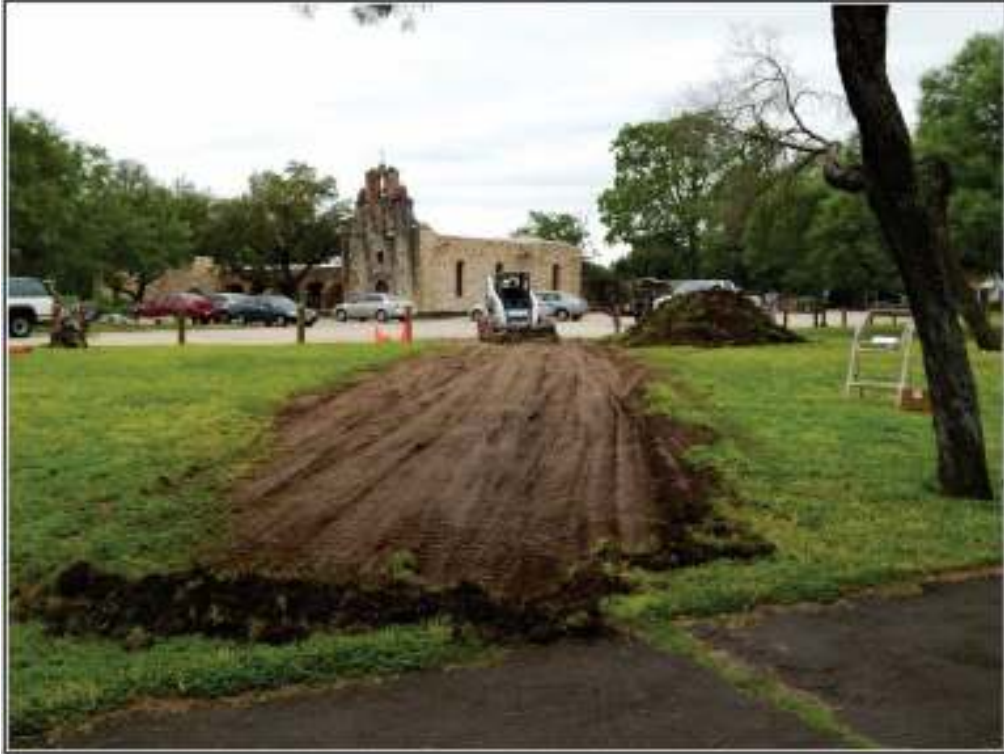
Figure 4-4. Completed swale with sloped edges.
