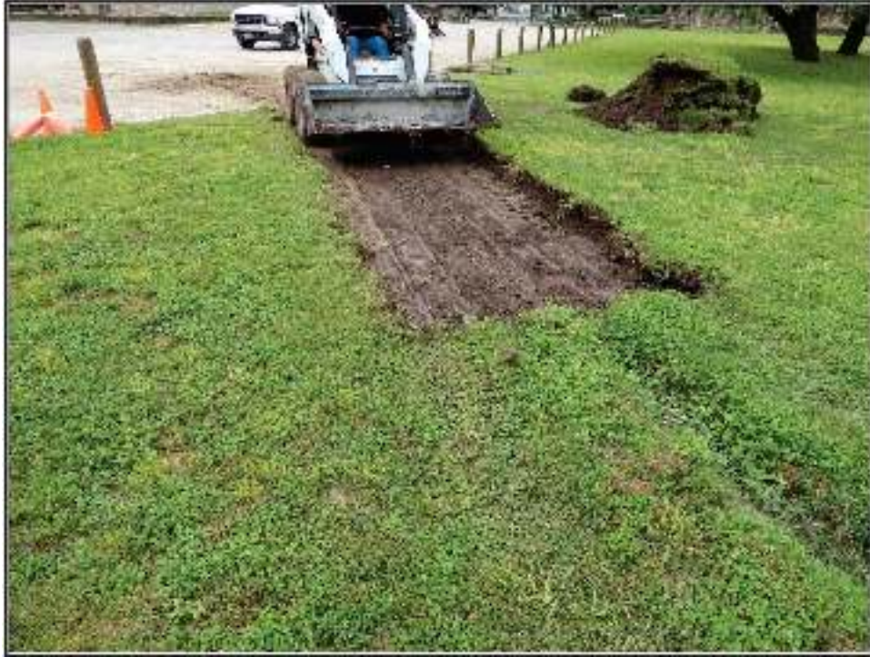
Figure 4-2. Recent swale enlargement centered on the existing swale.
