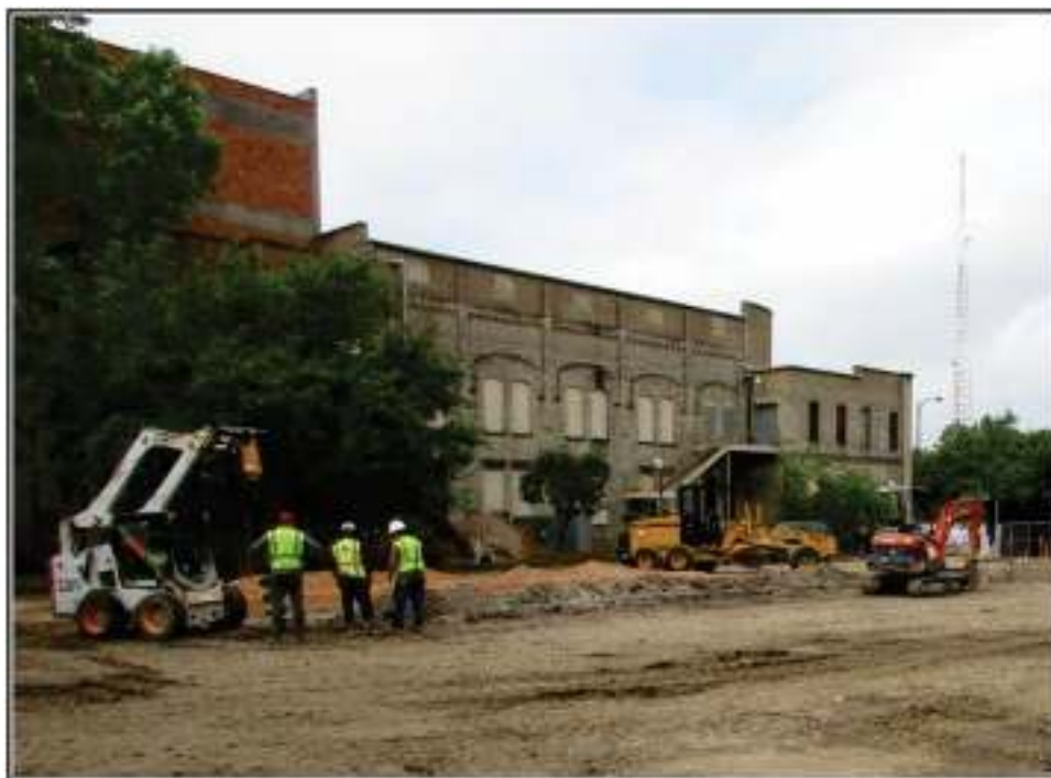
Figure 1-4. Electrical crew in the process of drilling a pier hole at the eastend, April 12, 2016. View to the southwest.
