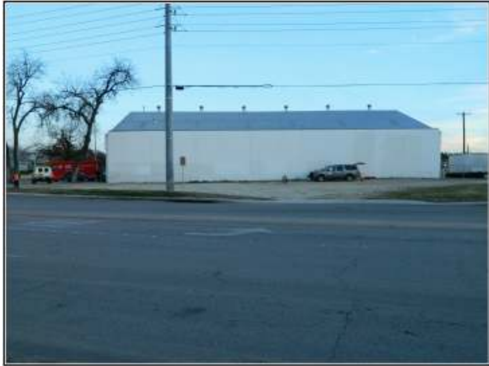
Figure 1-2. General view of the APE facing north.
