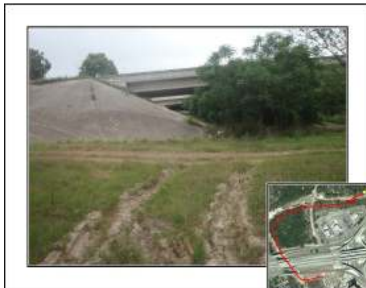
Figure 4-9. Two, two-track roads and IH-10 access road on eastern end of project area.
