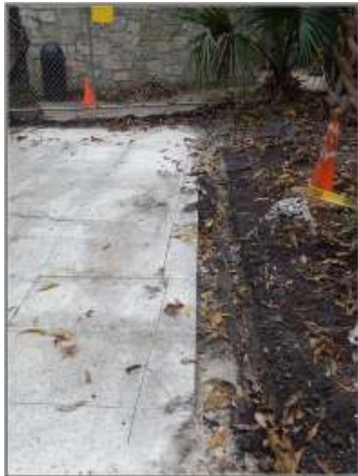
Figure 4-5. Trench for electrical conduit along first sidewalk before it was removed.
