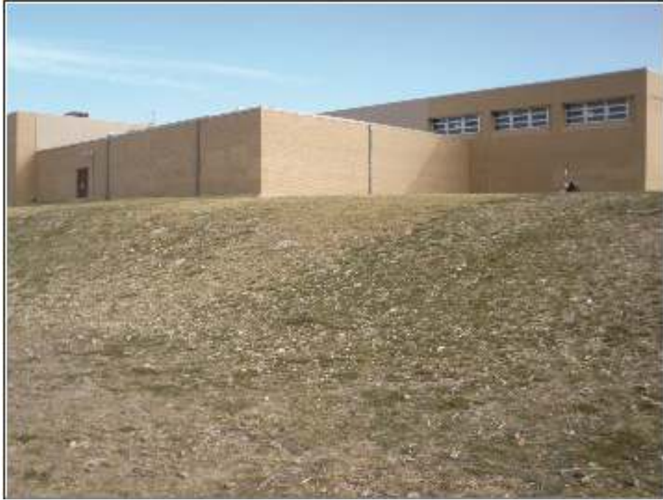
Figure 4-2. Disturbed area southwest of current YMCA building, showing eroding bedrock with ST 5 in background.
