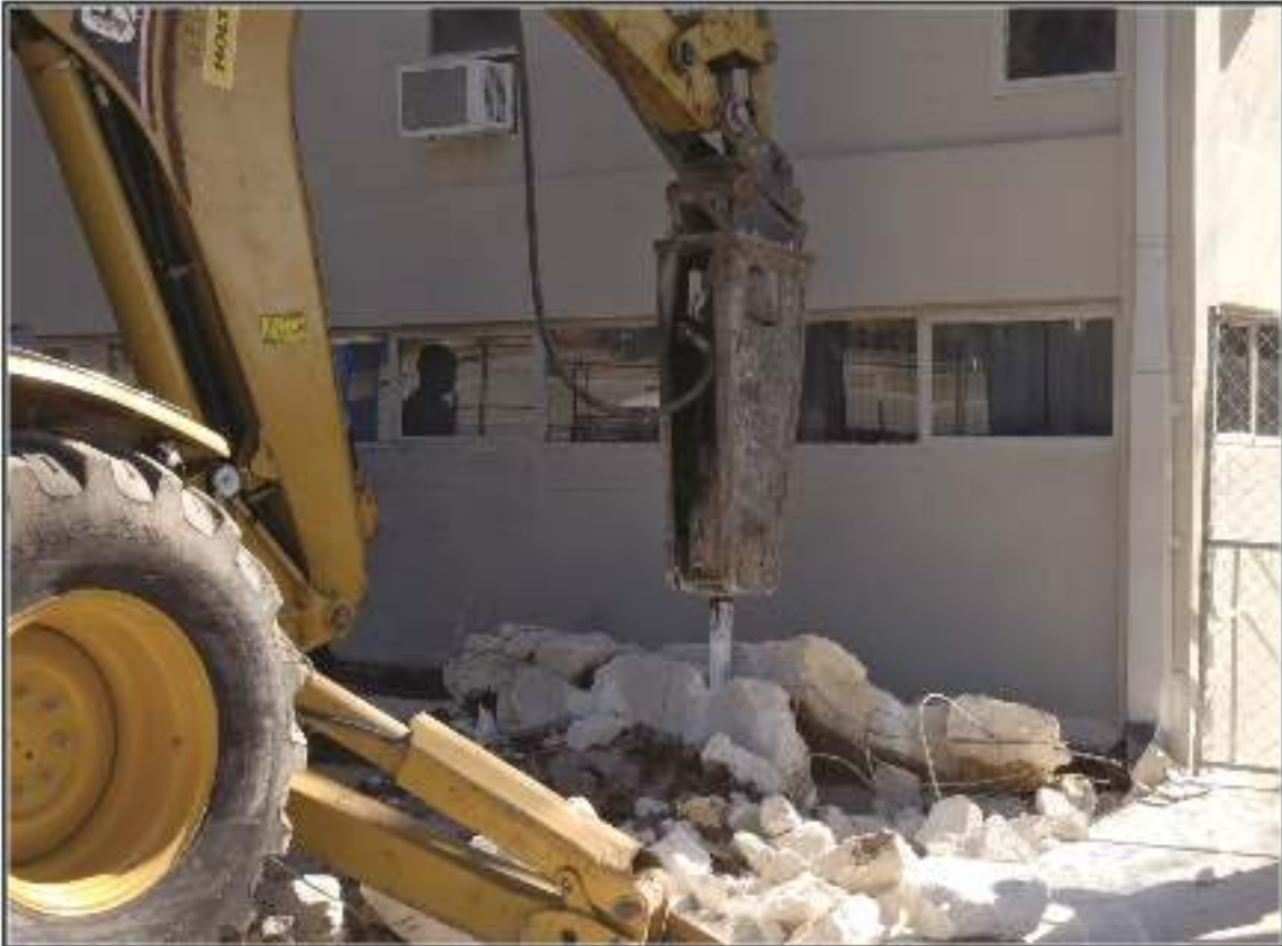
Figure 1-5. Demolition associated with the planned drainage improvements.
