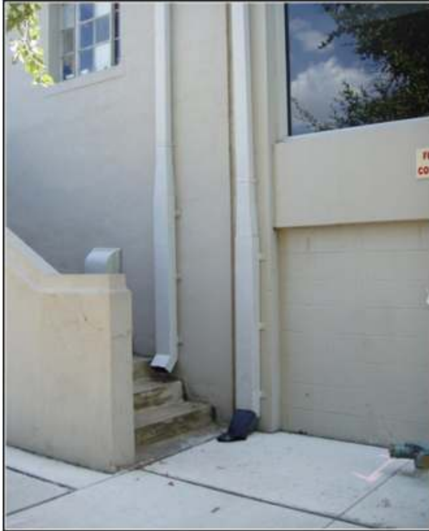
Figure 1-4. Close-up of two downspouts at the base of the stairs.
