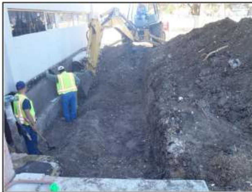
Figure 4-3. Trench 1 being excavated by backhoe and shovels.
