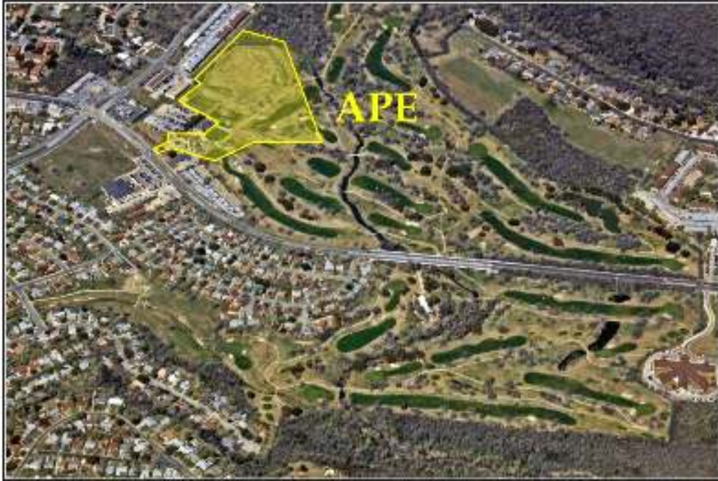
Figure 1-3. Project APE superimposed on the former layout of Pecan Valley Golf Club.
