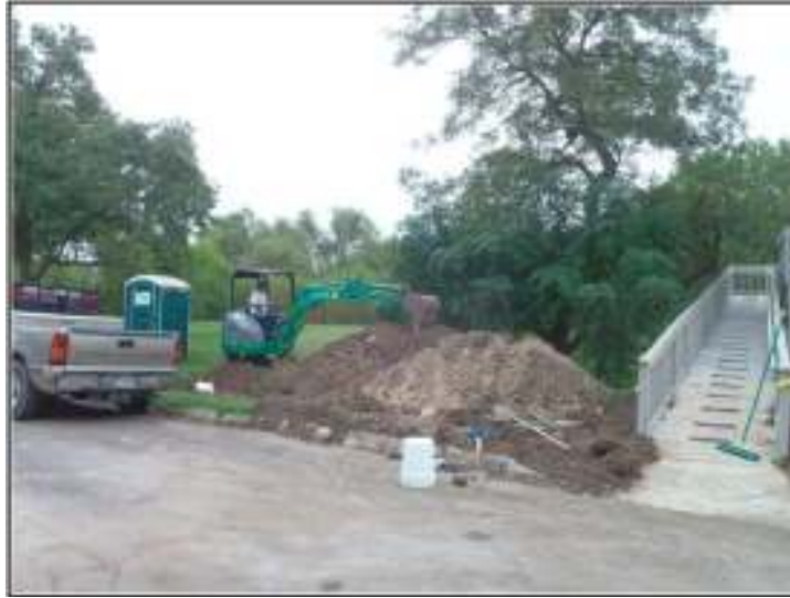
Figure 4-3. The excavation of Trench 2 near the southeast corner of Borglum Studio.
