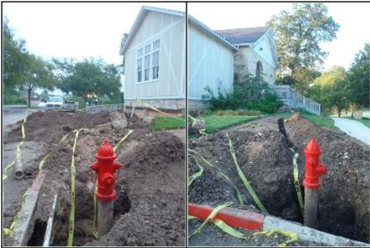
Figure 4-2. Excavation of Trench 1. Left side is prior to trench monitoring. Right side is hand excavated.
