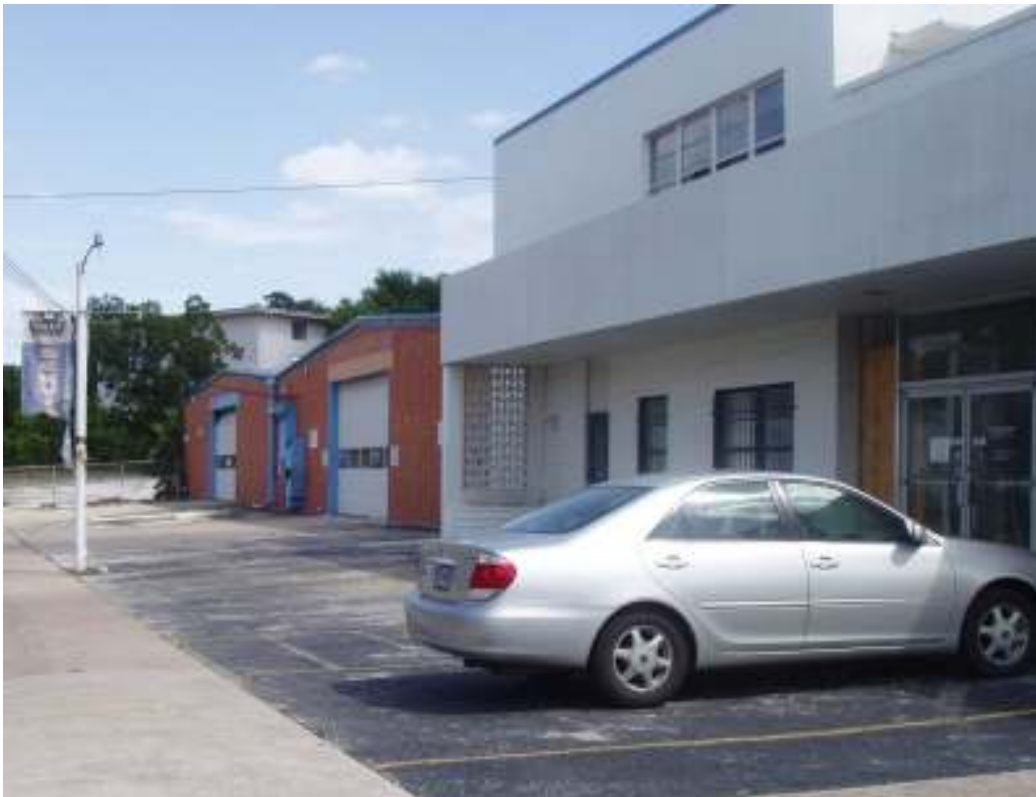
Figure 4-13. Brick body shops at back of dealership, looking east along Humphreys Ave.
