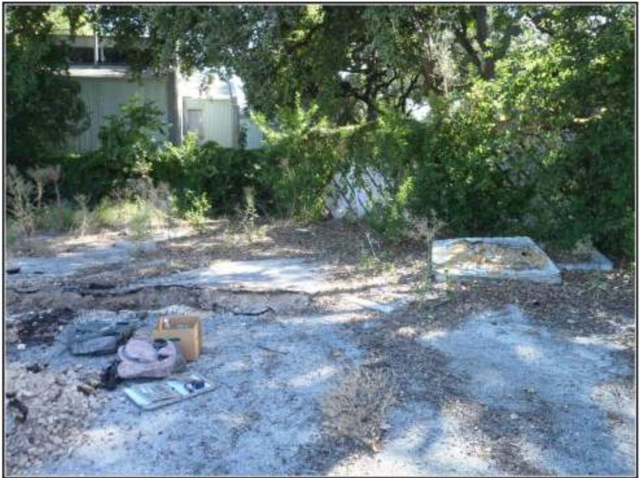
Figure 4-5. Location of BHT 2 and fill immediately below asphalt layer.
