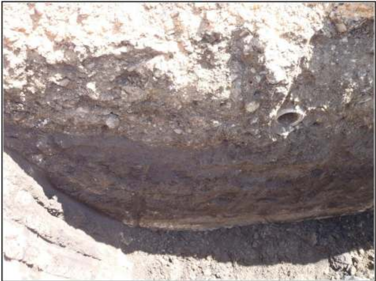
Figure 4-8. BHT 3, concrete pipe in north wall, note light caliche layer at the base of the trench.
