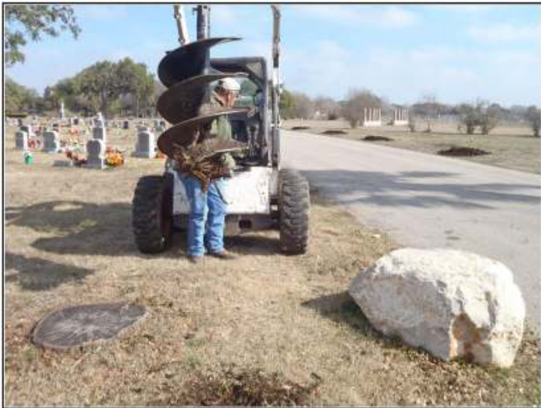
Figure 3-1. Bobcat mounted auger used to drill the planting holes.
