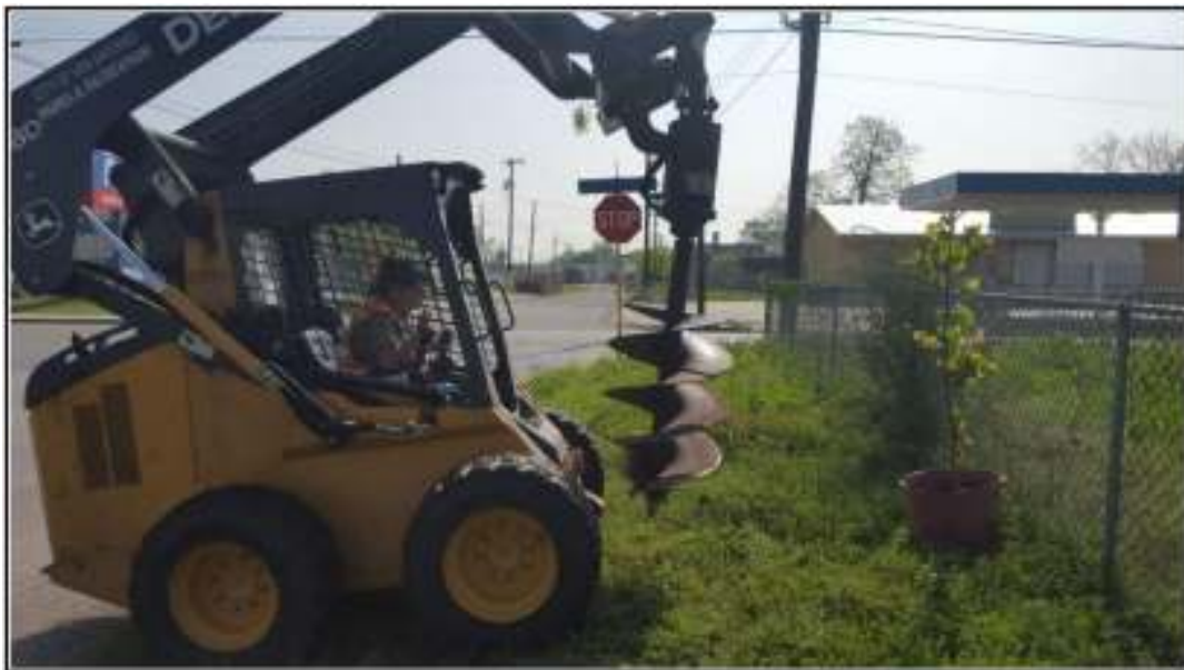
Figure 3-3. Auger boring at the City Cemeteries in 2015.
