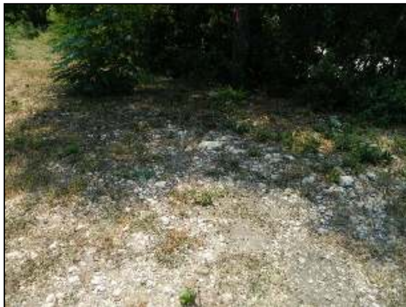
Figure 3-5. Exposed bedrock at the edge of the parking area, within the Area of Potential Effect.
