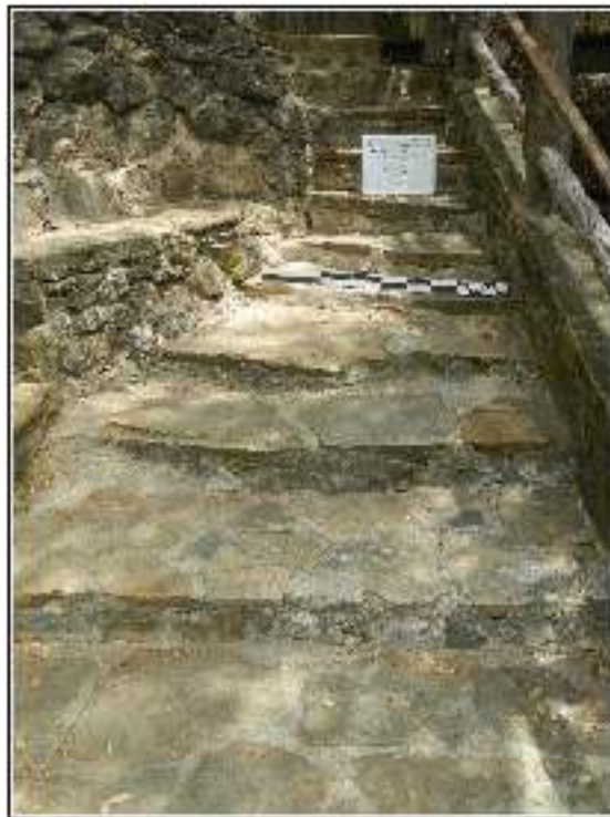
Figure 4-1. Stairs prior to initiation of demolition work by Frisch.
