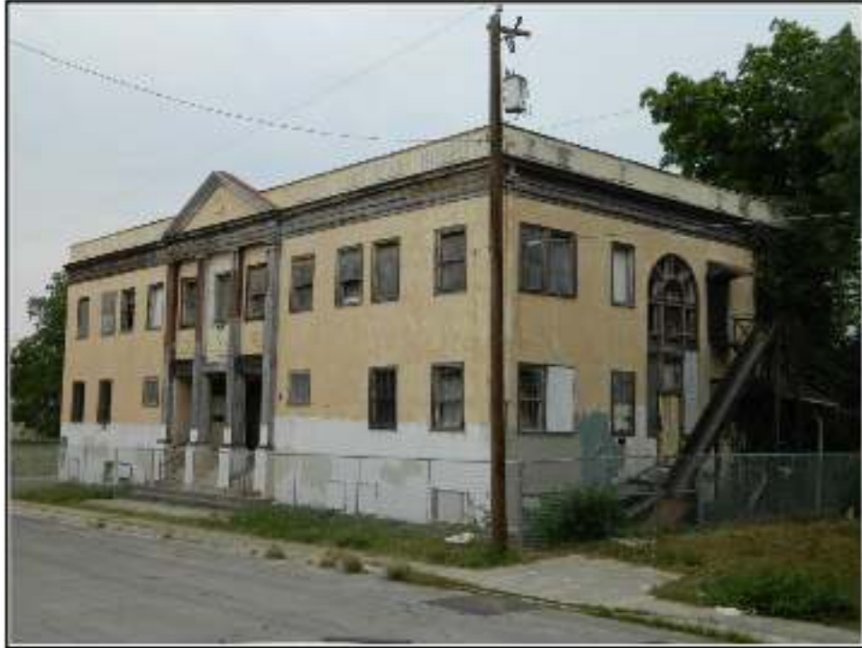
Figure 6-3. Historic Resource 1, the Good Samaritan Hospital.
