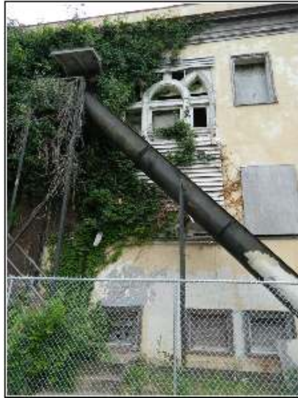
Figure 6-5. Window located on the north side of Historic Resource 1.
