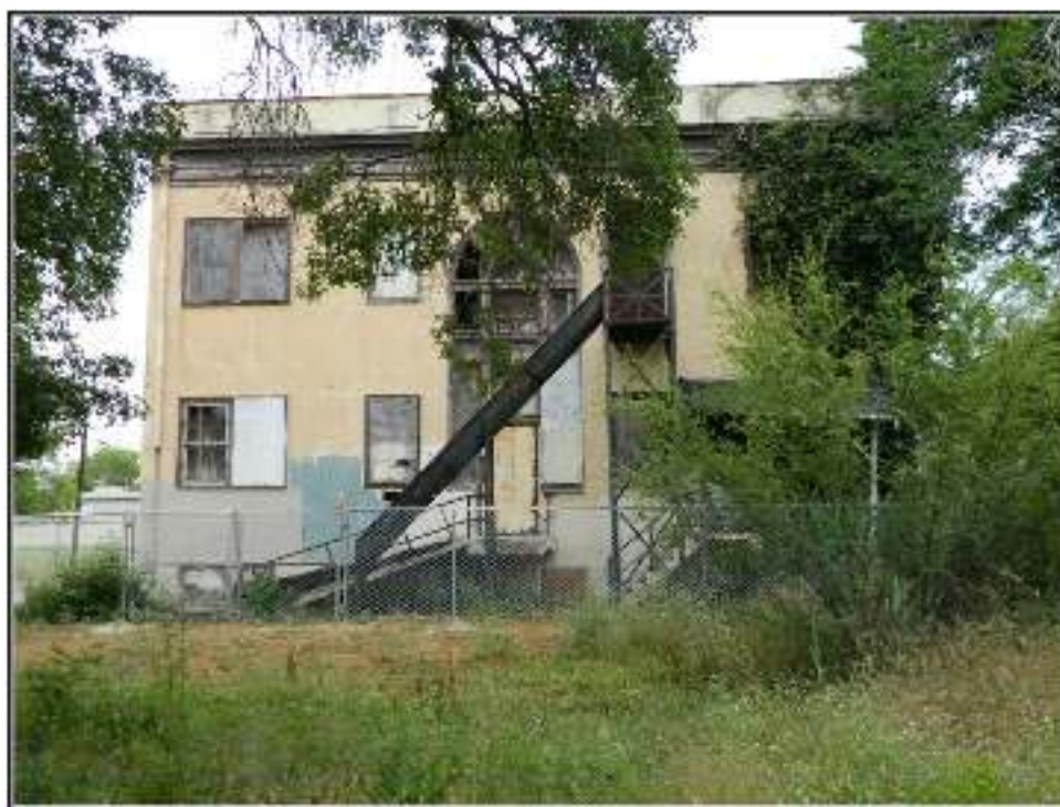
Figure 6-6. Metal fire escape slide located on the south side of Historic Resource 1.
