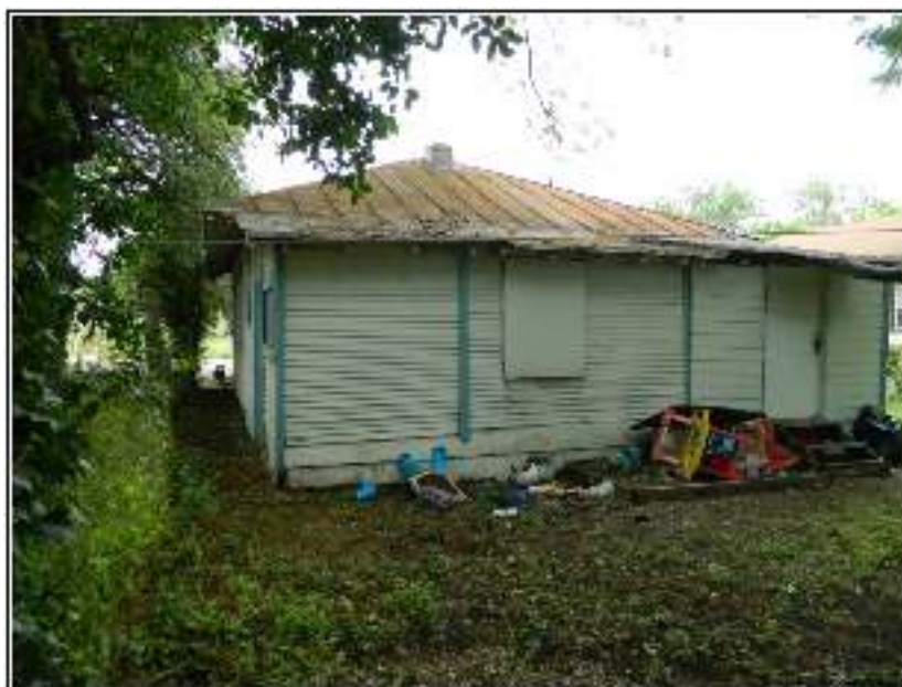
Figure 6-21. Historic Resource 3, south elevation.
