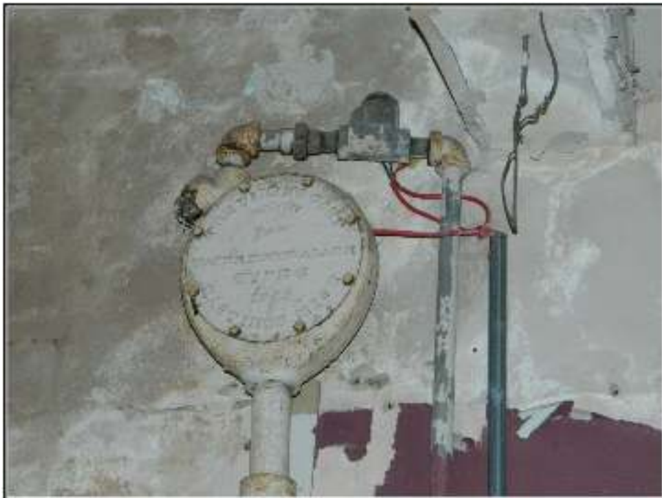
Figure 6-13. Water valve noted on the main floor of the northwestern room in the hospital.
