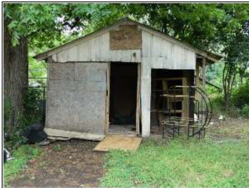
Figure 6-22. Associated structure located at the rear of the lot, Historic Resource 3.
