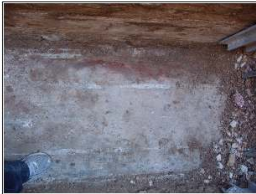
Figure 4-6. Concrete slab at the base of backhoe trench.
