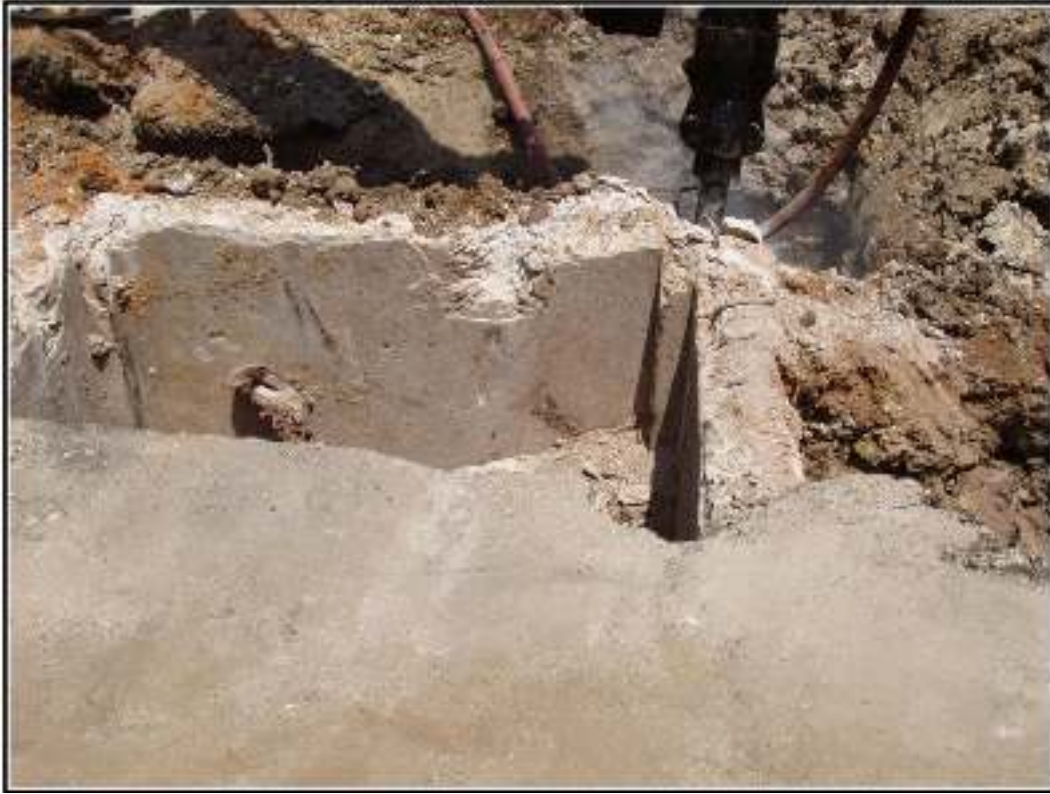
Figure 4-15. Elevator shaft exposed in T-5.
