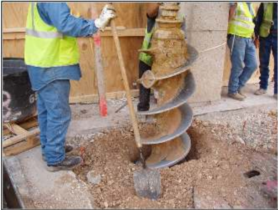
Figure 4-3. Auger bore excavation to determine the nature of the substrate.
