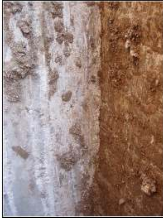
Figure 4-5. Concrete wall abutting brick wall at the west end of T-2.
