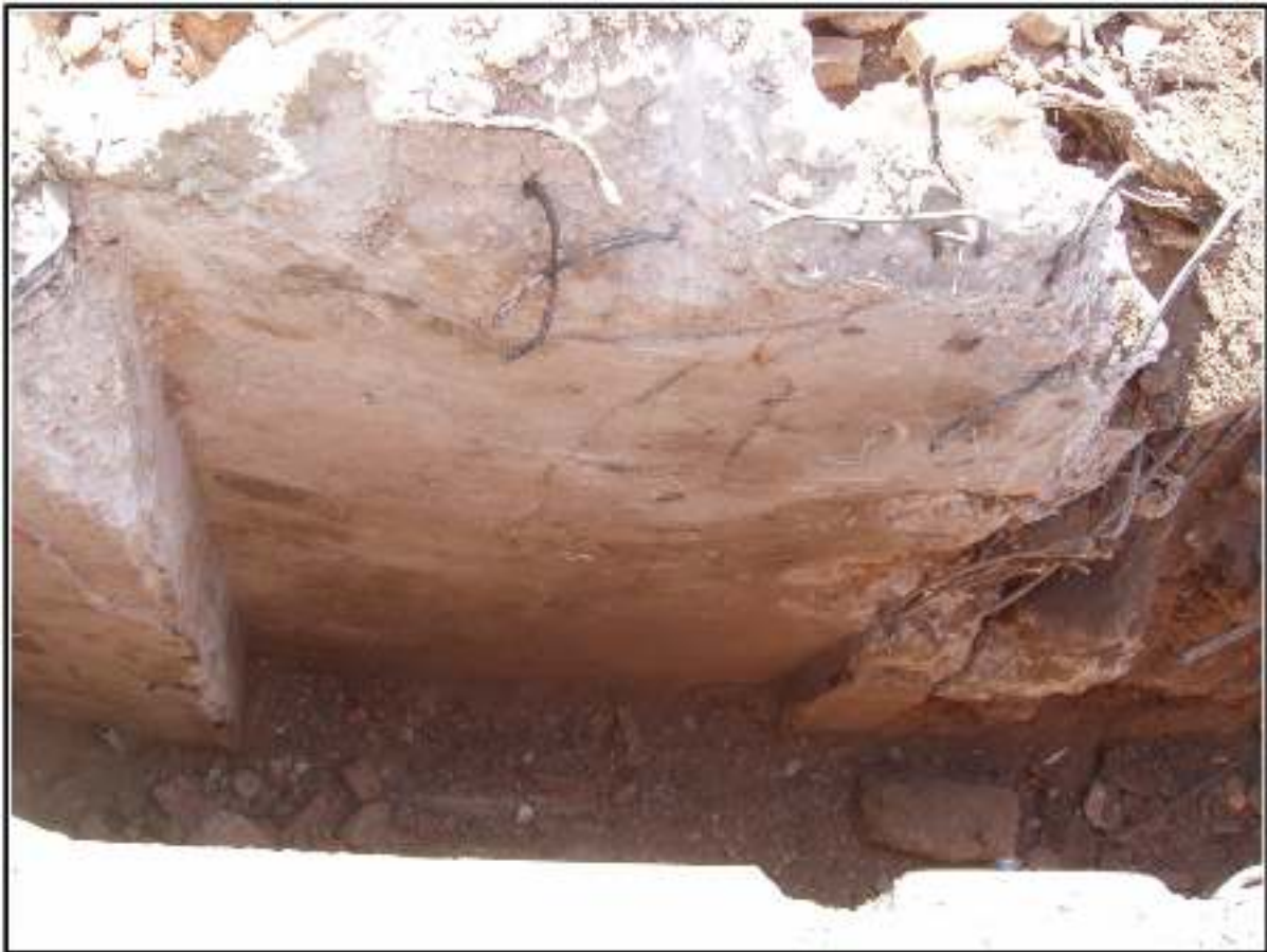
Figure 4-13. Reinforced concrete wall encountered in T-2.
