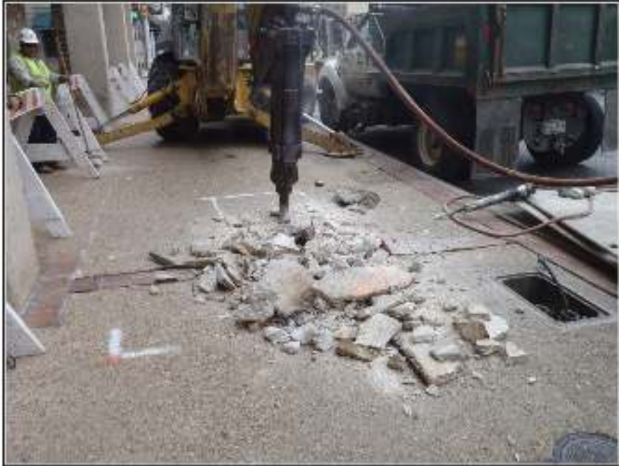
Figure 4-2. Removal of the sidewalk.
