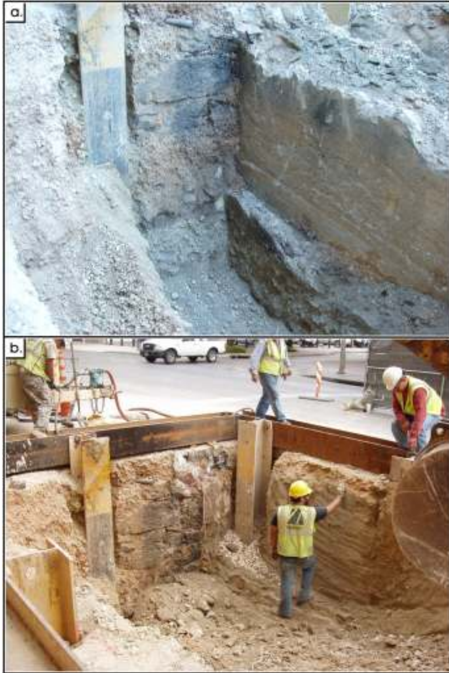
Figure 4-8. Western end of T-3: a) concrete wall abutting limestone blocks; b) note the continuation of limestone blocks beyond where concrete wall stood.
