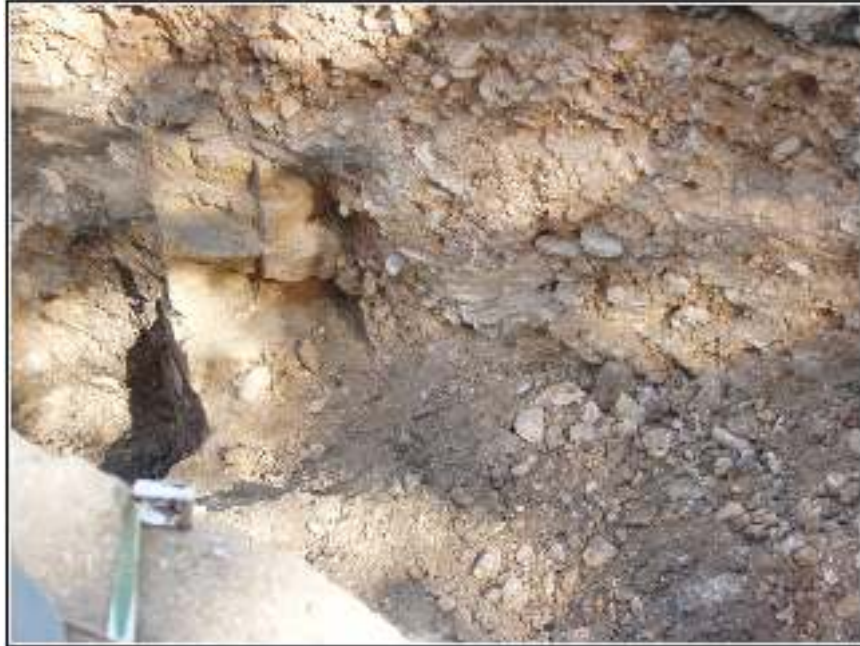
Figure 4-16. Sandstone wall in Manhole Trench 1.
