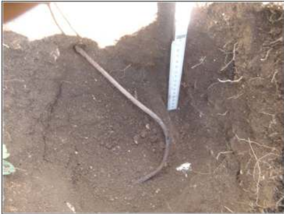
Figure 4-19. ST 7 at 30 cm (12 in.) with wire and PVC water line and valve. Well head is 5 m (16 ft.) south.
