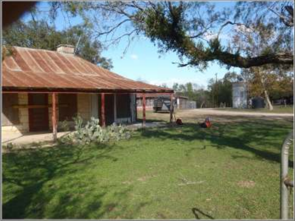
Figure 4-14. 41BX1744 stone house looking northeast towards driveway.
