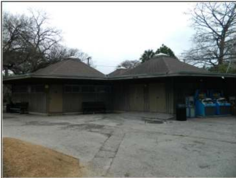
Figure 6-5. Historic Resource #4, larger building that houses the Wild Wonders exhibit.
