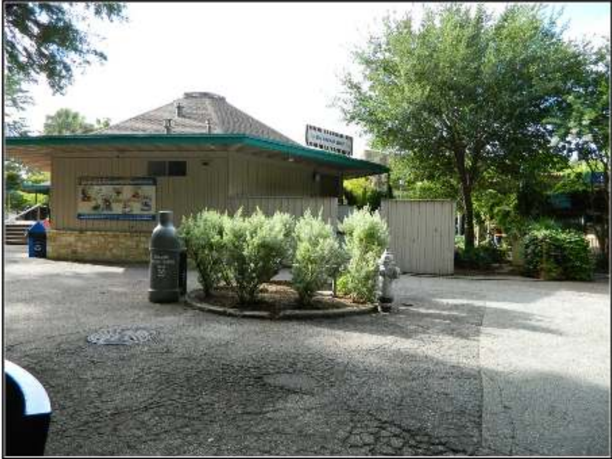
Figure 4-12. Culvert connecting sewer lines in the vicinity of the Ice Cream Shop.
