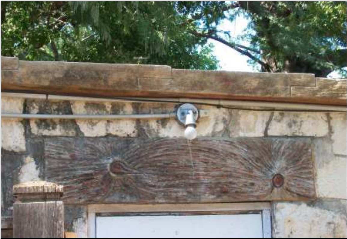
Resource #10 detail of faux bois lintel and “shingles”
