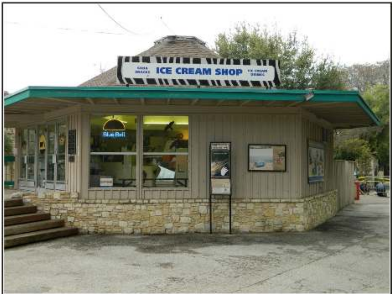
Figure 6-2. Historic Resource #1, the Ice Cream Shop located next to the Tiny Tot Nature Spot at the San Antonio Zoo.
