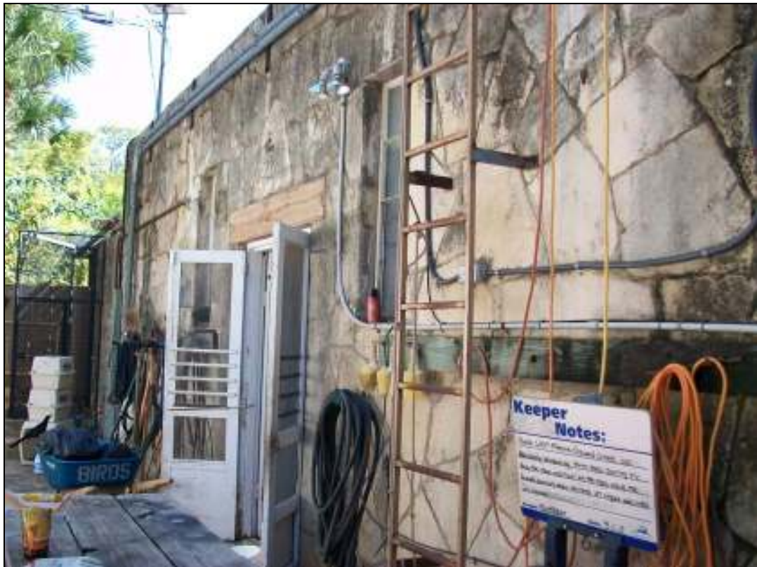
Resource #8 – rear elevation with casements and faux bois lintel
