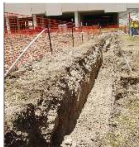
Figure 4-3. SpawGlass Trench 2. Note utilities exposed in walls.
