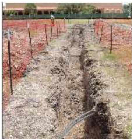
Figure 4-2. SpawGlass Trench 1. Note utilities exposed in walls.
