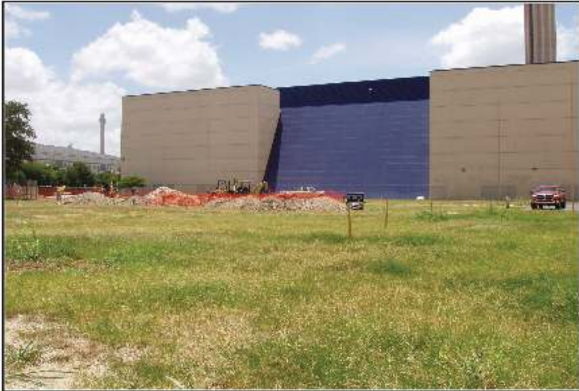
Figure 1-3. Overview of the APE looking southeast toward the Convention Center. Stakes mark a buried water line.
