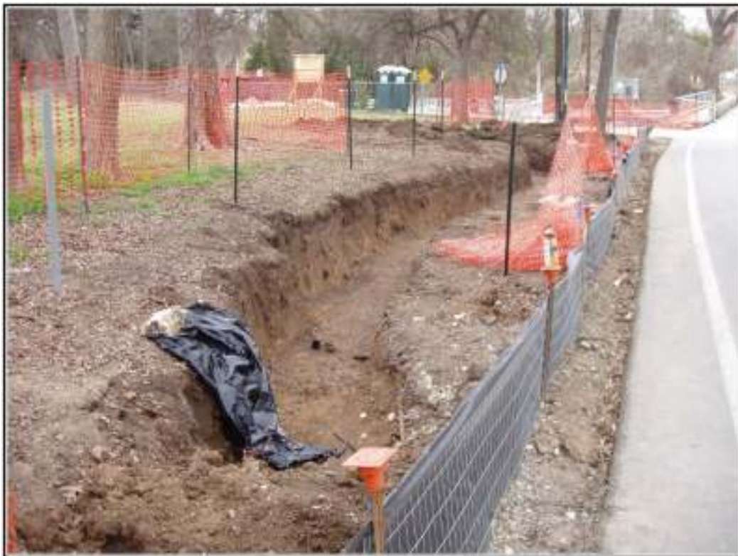
Figure 2-1. Retaining wall trench south of Mulberry Avenue.
