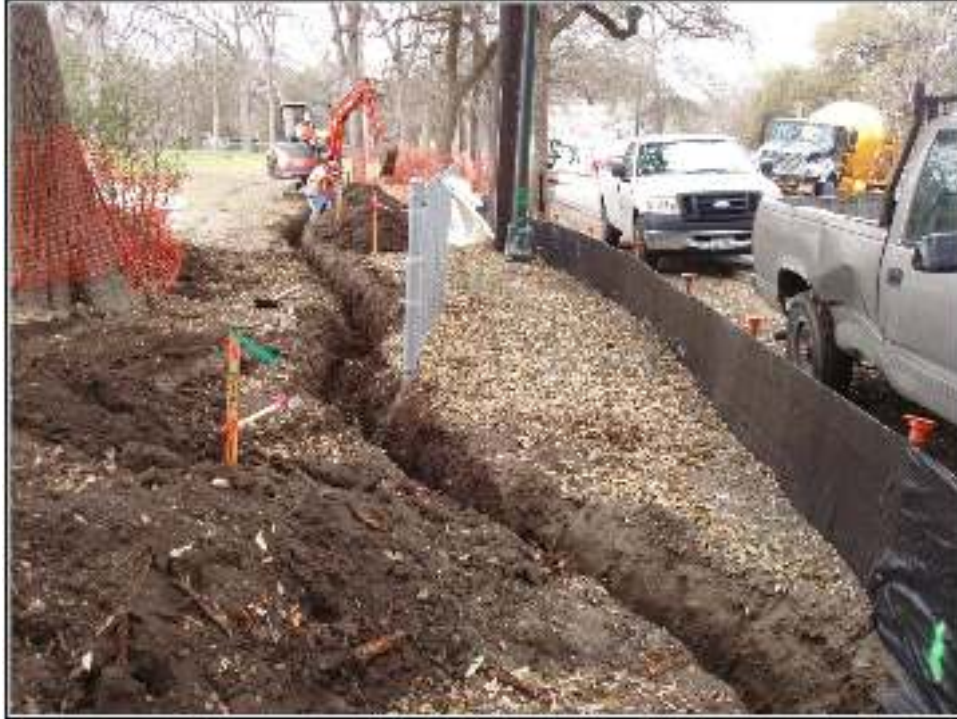
Figure 2-2. Utility trench connecting light poles along sidewalk.
