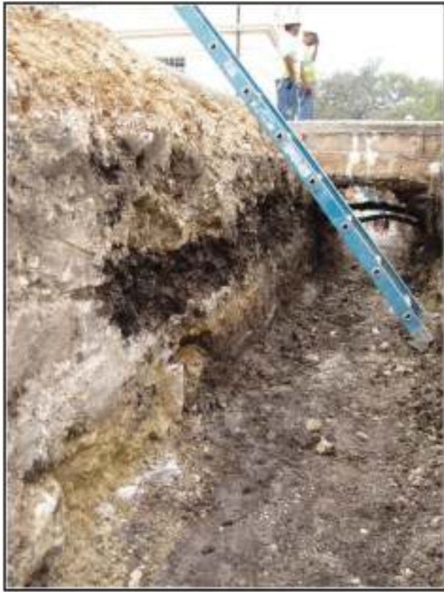
Figure 3-5. South wall profile of the fire/water line trench showing successive layers of modern fill materials.
