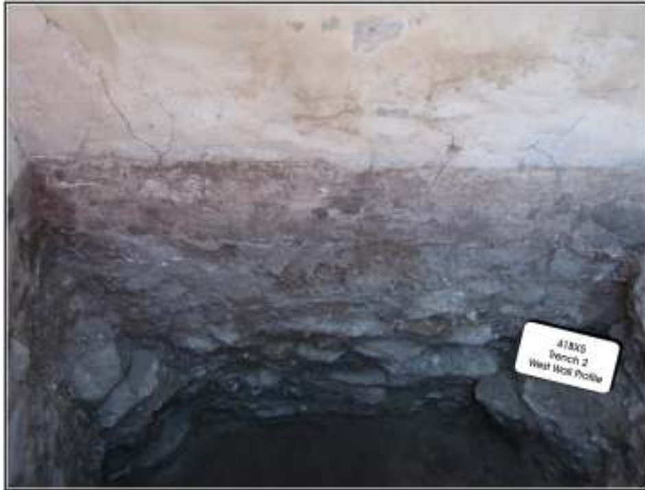
Figure 3. West wall of Trench 2 showing the wall and foundations exposed in the current re-opening of the trench.
