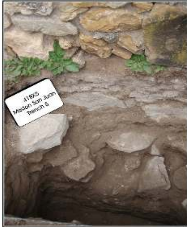
Figure 10. Trench 5 view of foundation and electrical cable (lower left corner).
