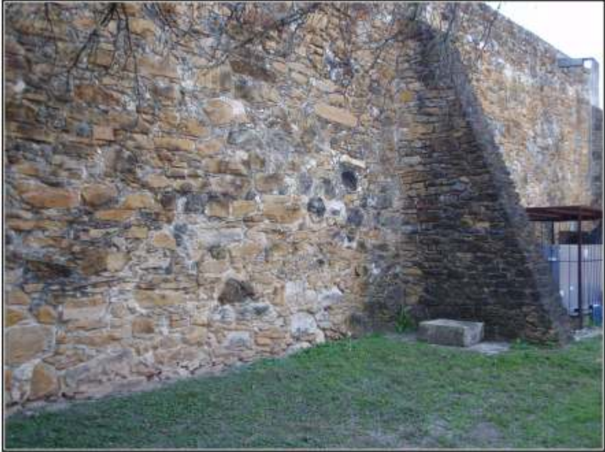
Figure 8. Western wall of church showing the location of Trench 5 and the stone drainage feature obstructing the southern part of Trench 5.
