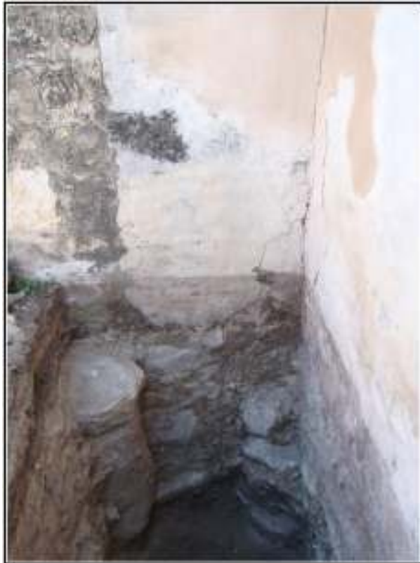
Figure 5. Overview of the south wall of Trench 2 showing the wall of the buttress and foundation.
