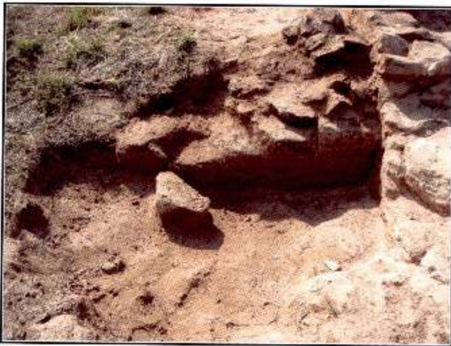
Figure 16. The eastern façade of the northern portion of the wall dividing Rooms 1 and 2, facing west.
