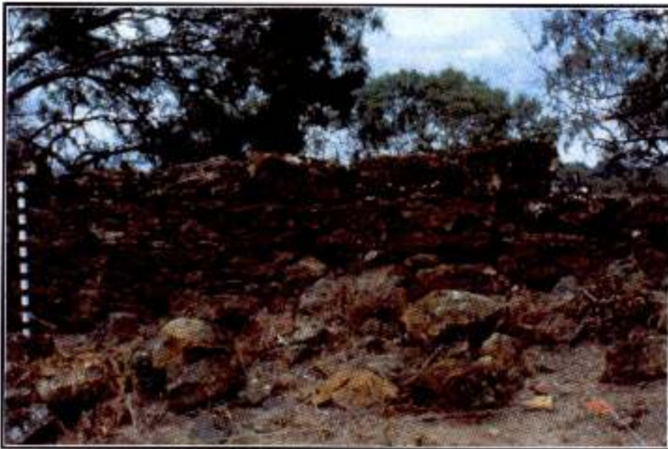
Figure 5. The south side of the north wall of Room 1 taken during the 1980s, facing north.
