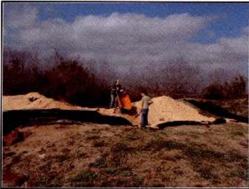
Figure 26. Backfilling with sand using shovels and wheelbarrows.
