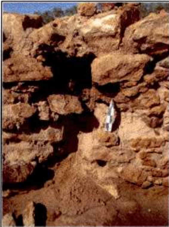
Figure 24. Sand washed out from between the building stones along the north wall of Room 1.
