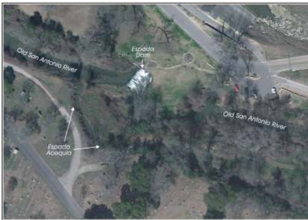
Figure 1-5. Aerial view of Espada Dam and the beginning of the Espada Acequia, a design very similar to the San José Dam.
