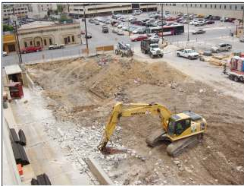
Figure 4-8. Demolition of low wall on northern portion of APE.
