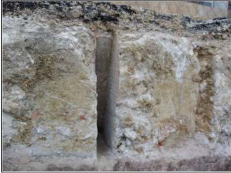
Figure 4-3. Slots in dry goods warehouse foundation.
