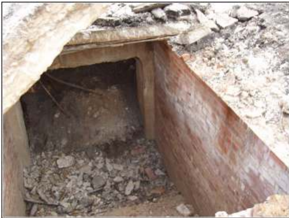
Figure 4-16. View of room adjoining dry goods warehouse basement.
