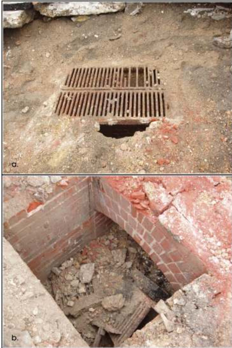
Figure 4-14a, b. Views of red brick drain.
