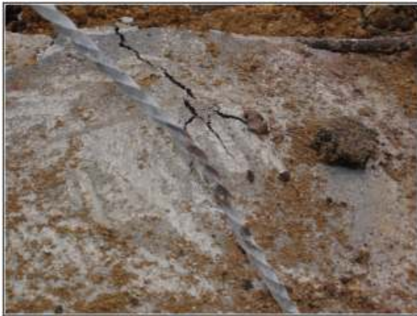
Figure 4-4. Spiral rebar sample.
