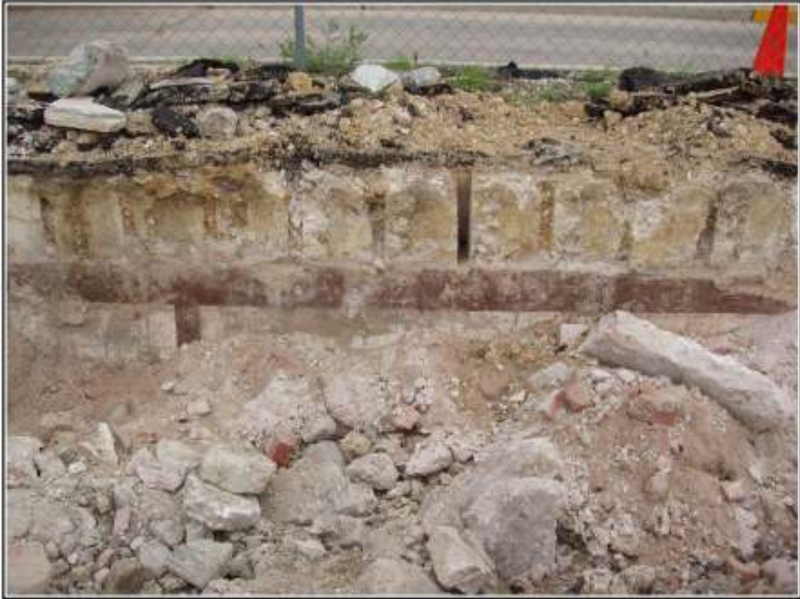
Figure 4-2. Dry goods warehouse foundation and fill. Note red/brown stripe near top of foundation.
