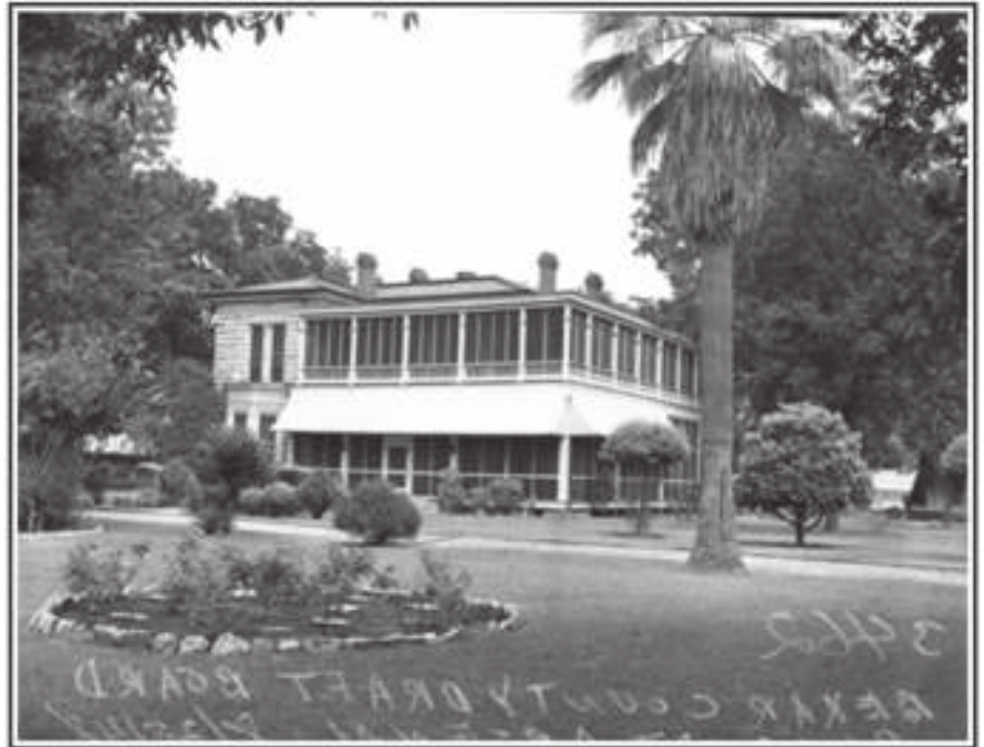
Figure 2-4. Photograph of the Commanders House taken in 1948. Note that the balconies have been enclosed (Photograph is in the collection of the Institute of Texan Cultures, #L-6432-F).
