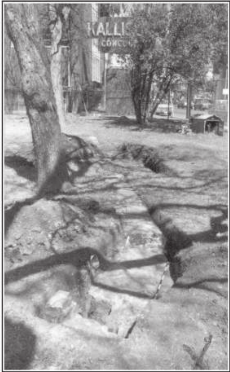
Figure 1-3. Photograph of the west wall of the San Pedro Acequia on the grounds of the Commander's House taken during excavation by CAR, showing curve of the acequia and a gate to a lateral that led west (foreground). Facing North.
