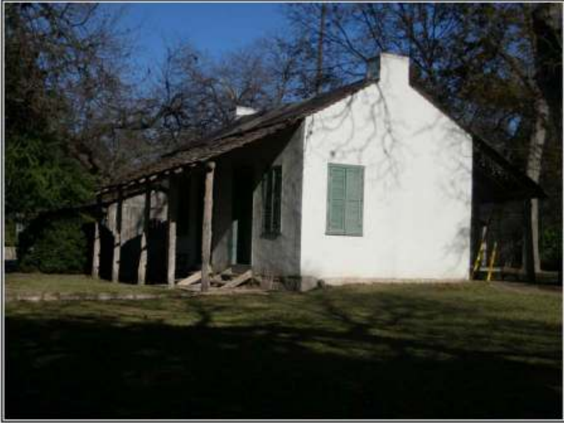
Figure 4-4. Photograph of the Navarro House.
