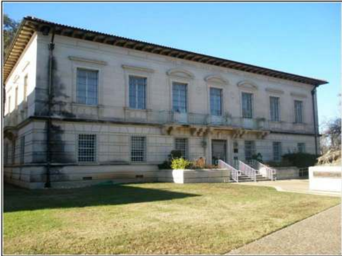
Figure 4-6. Photograph of the Pioneer Hall.
