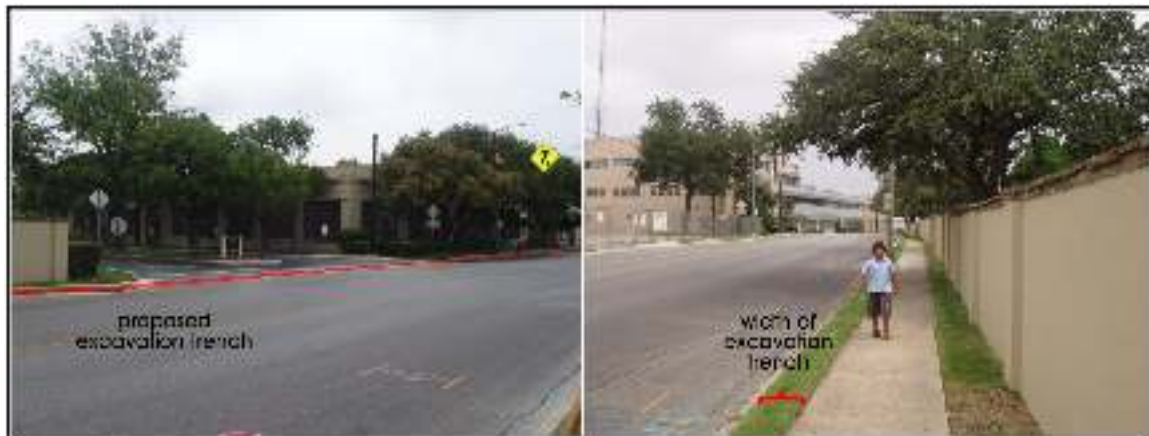
Figure 3-1. Photograph (left) shows main entrance to HFB headquarters and length of excavation in red. Photograph of project area along S. Main Avenue with the width of excavation trench (right).
