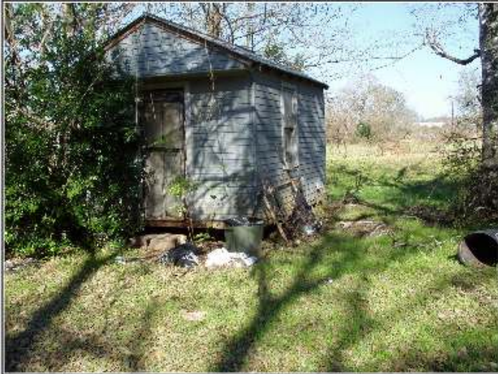
Figure 4-4. Only remaining structure at location of 1312 Farm Road.
