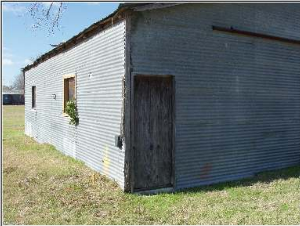
Figure 5-5. Undocumented structure in Block 53.
