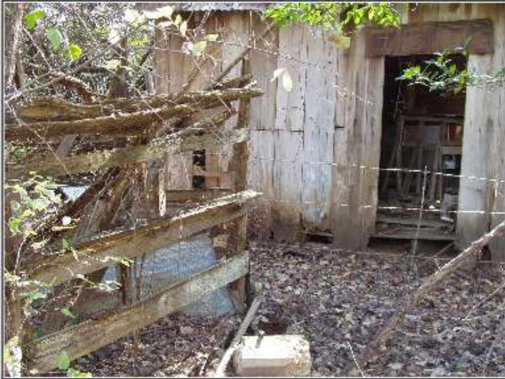
Figure 5-6. Undocumented structure in Block 70.
