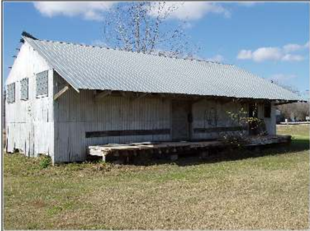
Figure 5-2. Undocumented structure in Block 53.
