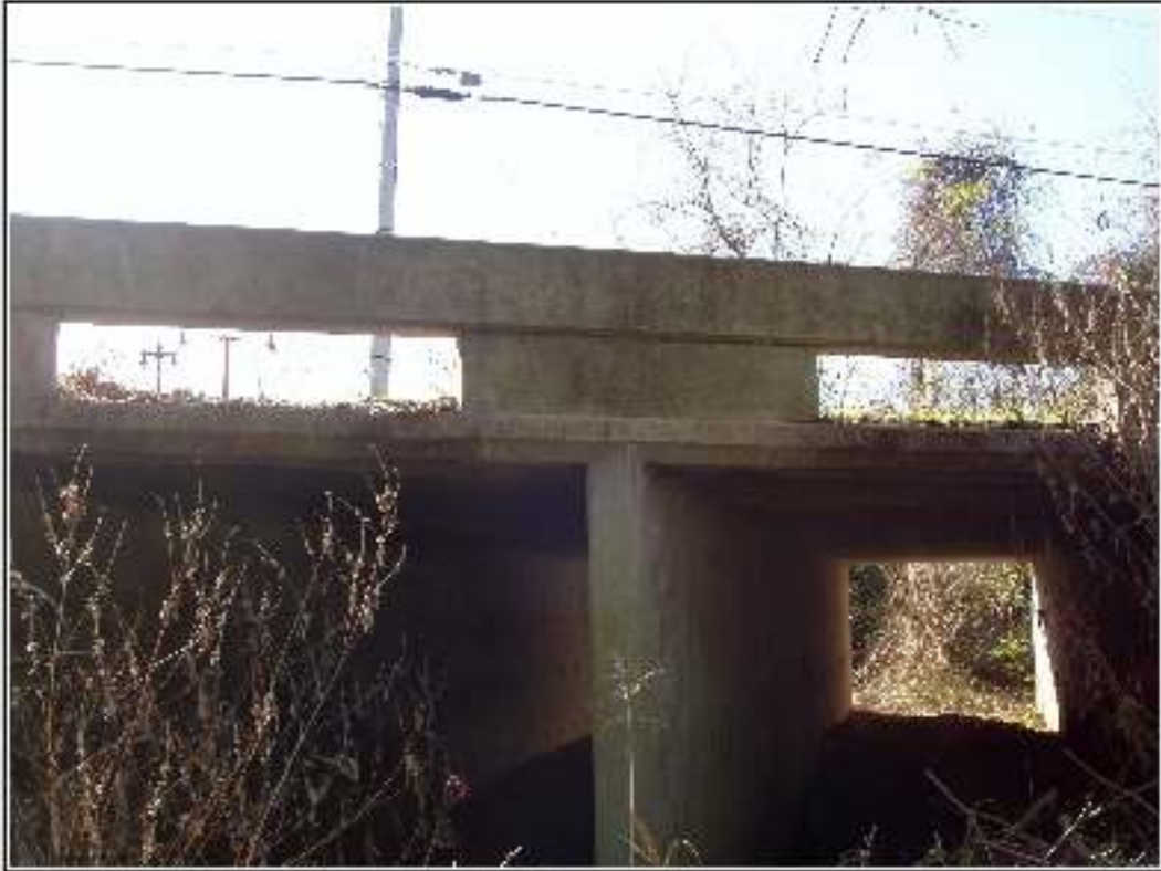
Figure 4-1. Closet bridge over Piney Creek.
