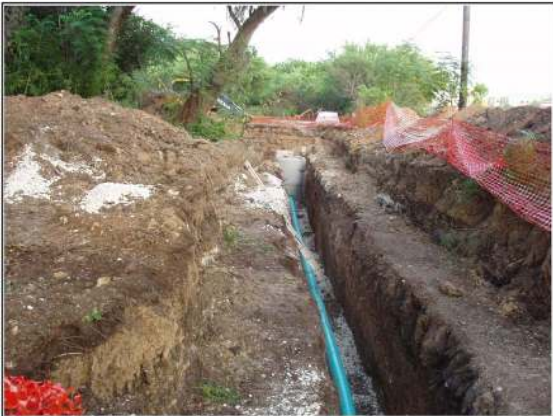
Figure 1-3. Utility trench across 41BX217.
