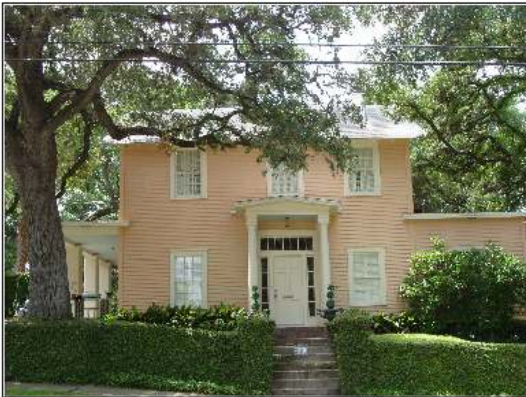
Figure 3-7. Photograph of the Nan Weinert Residence.
