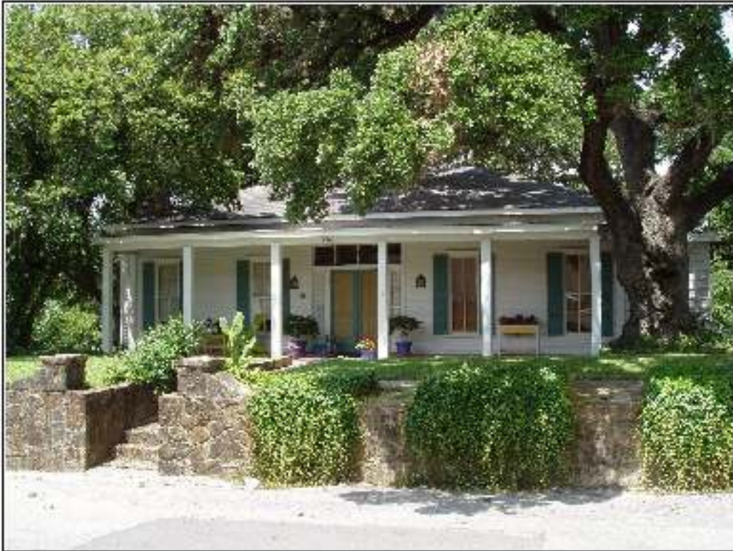
Figure 3-10. Photograph of the Robert Hall House.
