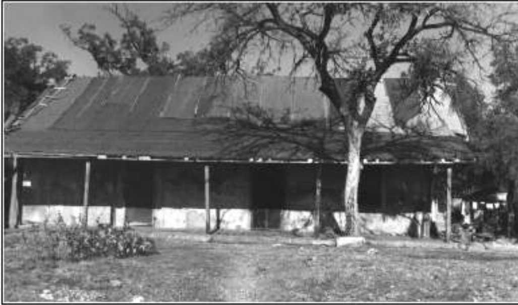
Figure 3-19. Photograph of the front of the Ranger Station.
