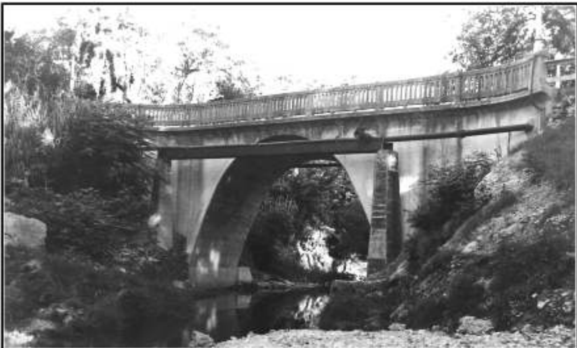
Figure 3-23. Photograph of the Nolte Street Bridge ca. 1935.
