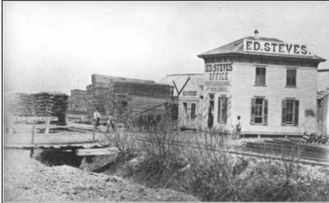
Figure 1-4. Photograph of Steves Lumber Company in 1881 with the Valley Ditch crossing diagonally in the foreground (photo courtesy of the Witte Museum, San Antonio, Texas).
