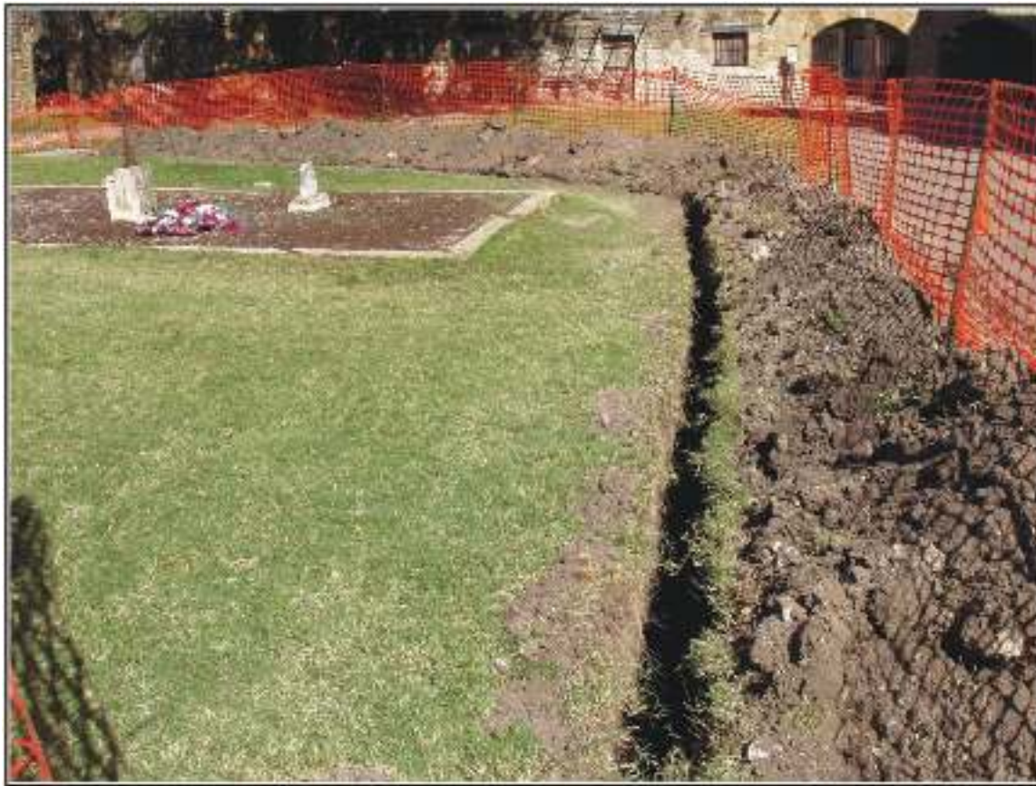
Figure 4-3. Photograph of the trenching past the cemetery. Facing northwest.
