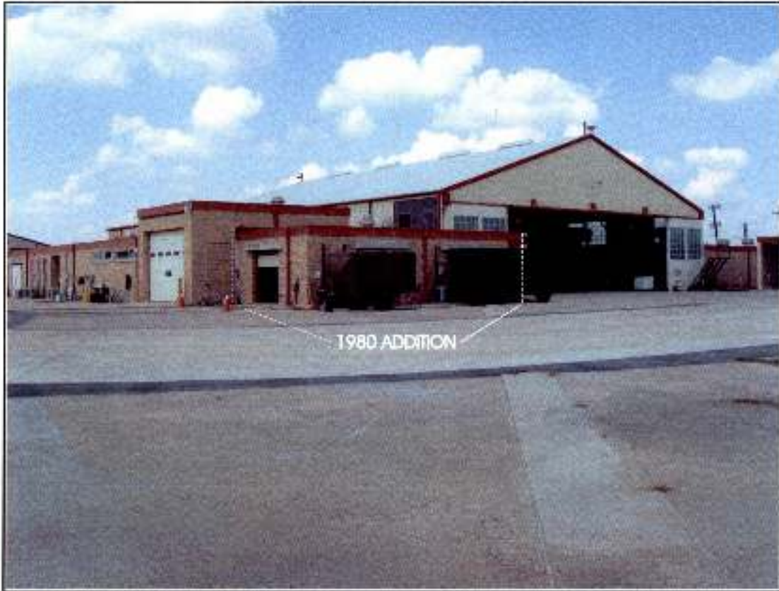
Figure 4-16. 2006 Photograph of the southeastern corner of the hangar added in 1980.
