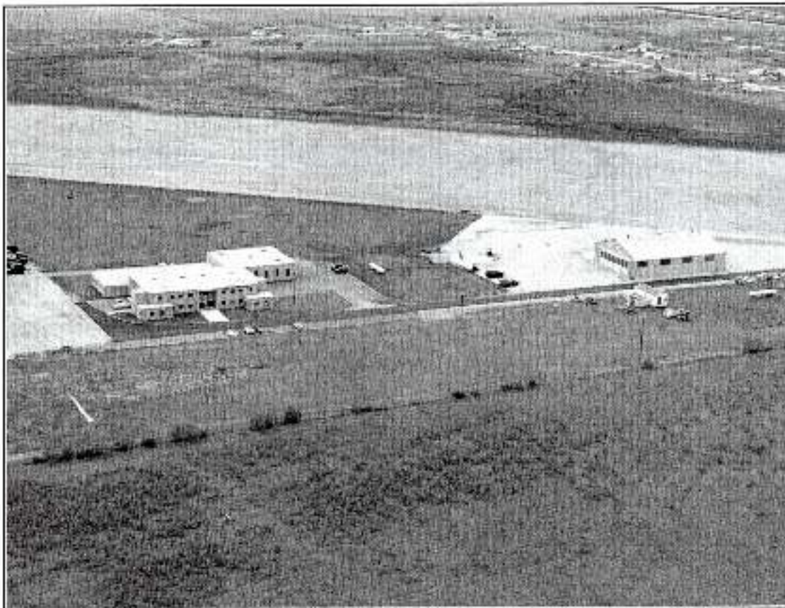
Figure C1. Aerial of Martindale Airfield showing Armory (left) and Hangar (right), view southeast. (Official Photograph Air National Guard Group 149th Fight Group, Kelly AFB, Texas. NEG #TANG 13 13 6).
