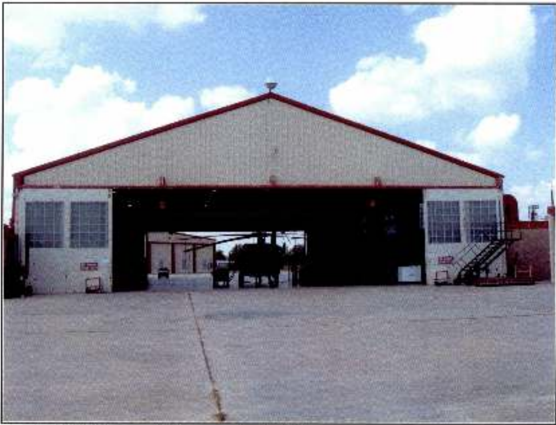
Figure 4-7. 2006 photograph of the eastern façade of the hangar.
