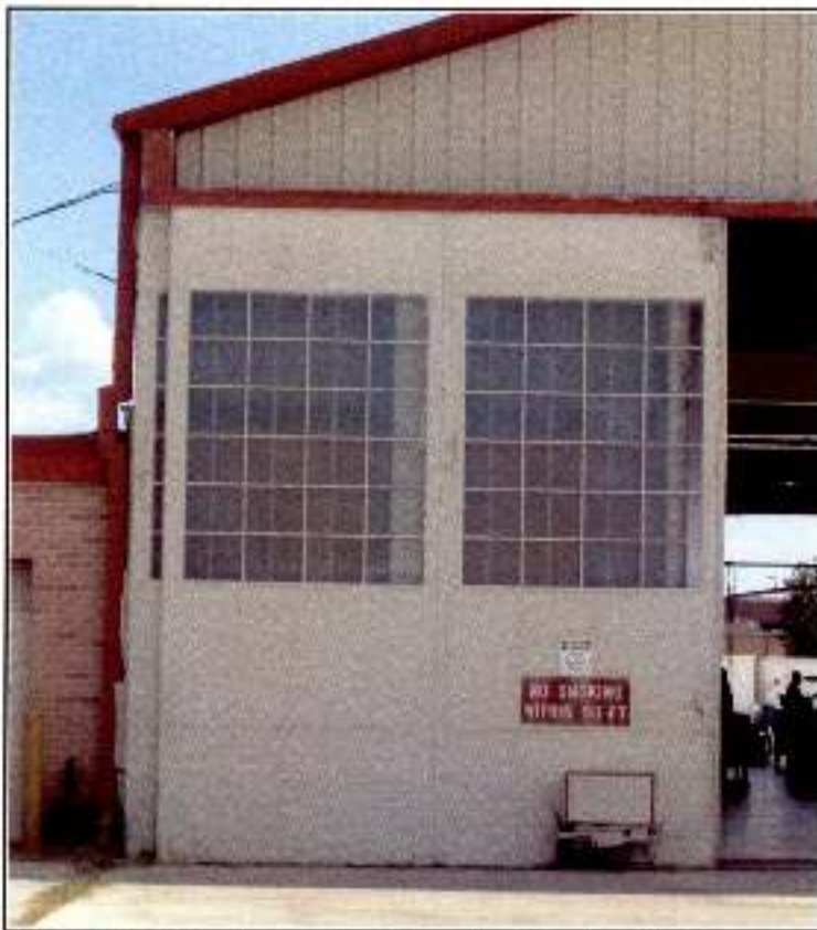
Figure 4-6. 2006 photograph of the western façade of the hangar, showing sliding doors.
