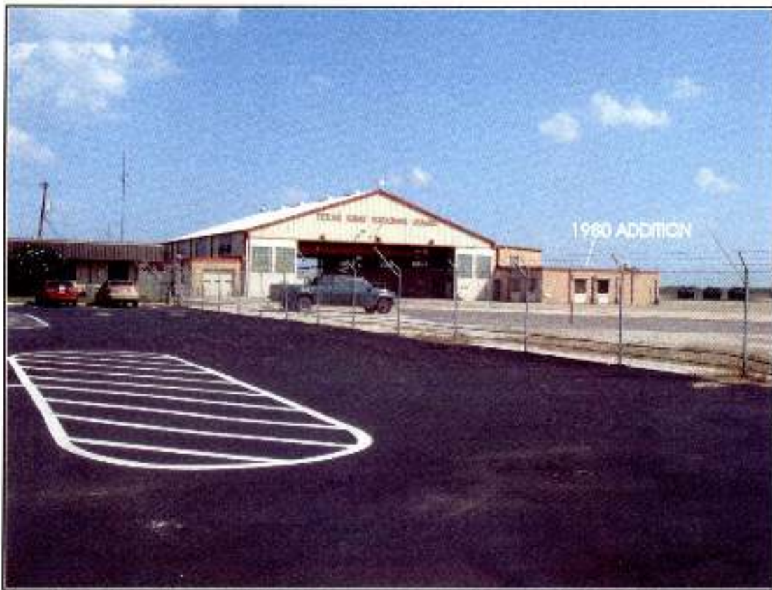
Figure 4-17. 2006 Photograph of the southwestern corner of the hangar added in 1980.
