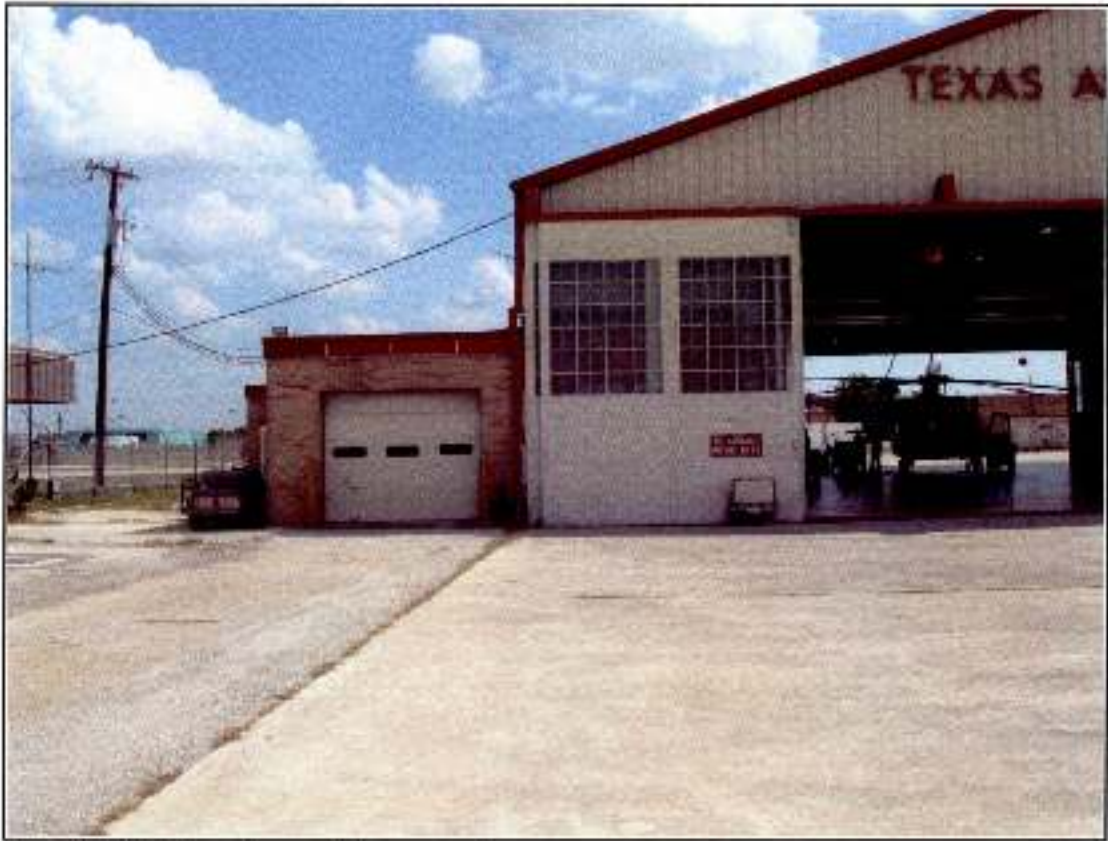
Figure 4-14. 1975 northern addition garage door, view east.
