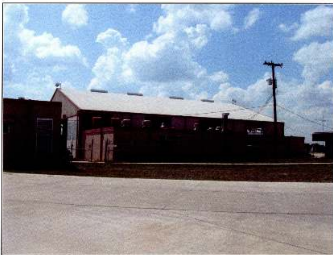
Figure 4-13. Northern addition to the hangar, built in 1975 (view south).
