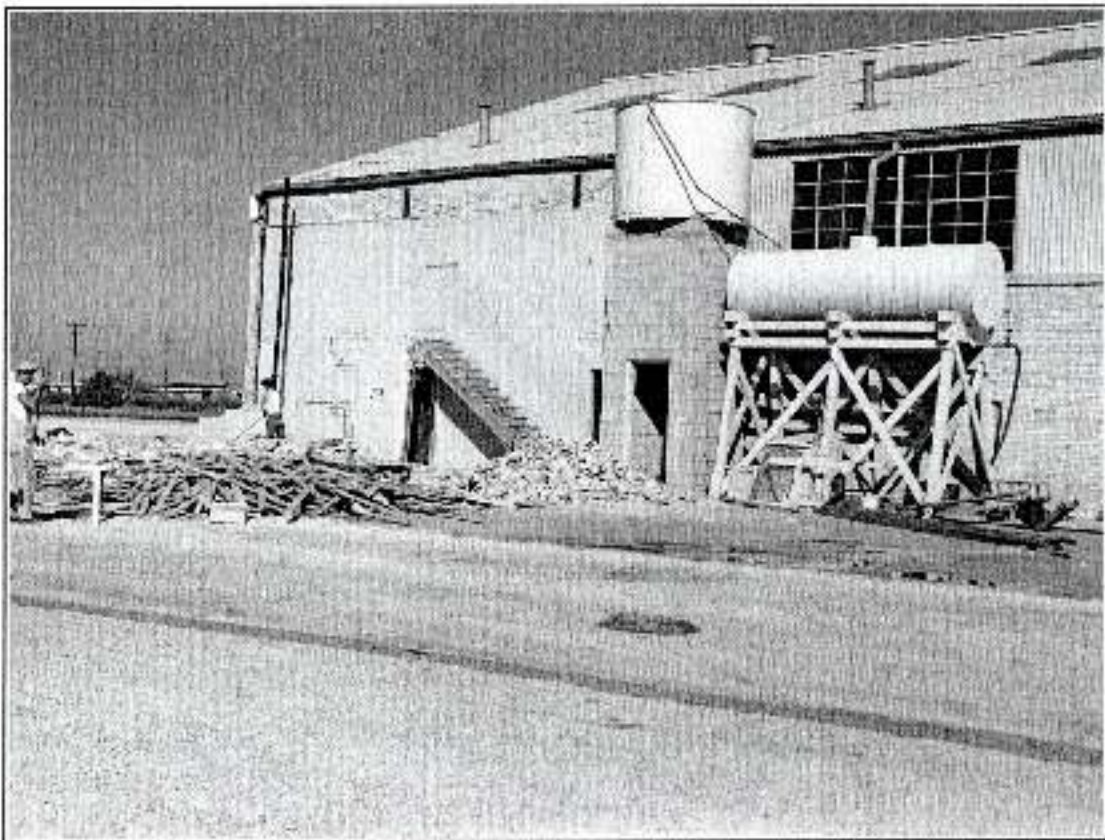
Figure 4-9. Cleanup efforts after the 1961 explosion in the southern annex of the structure show little damage to the main hangar, though six individuals were injured. Photograph by Sgt. Joe T. Elsis, TEXANG, 149th Fighter Group, Kelly AFB, San Antonio, Texas.
