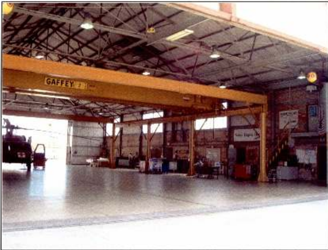
Figure 4-8. View inside the hangar of the modern "Gaffey" hoist system installed in the 1990s.
