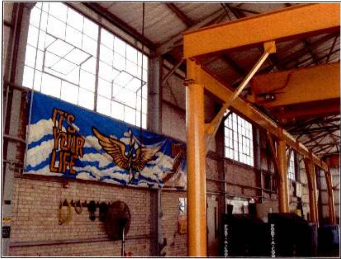
Figure 4-4. Hangar interior detail of windows.
