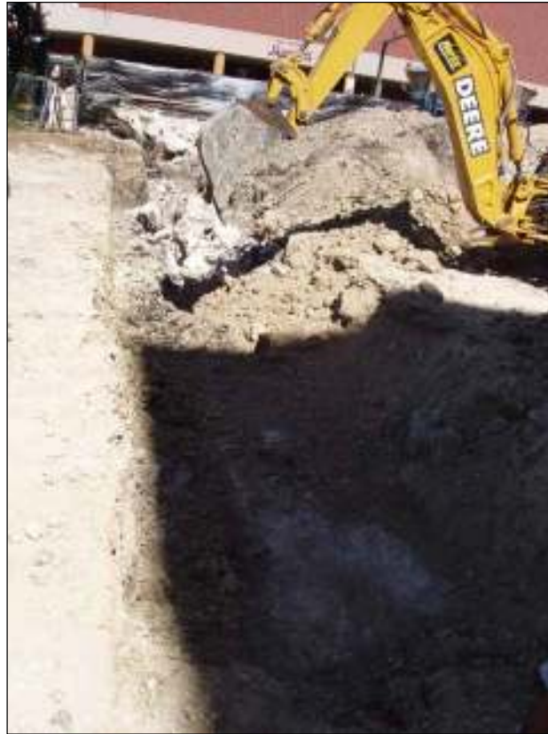
Figure 3-2. Photograph of mechanical excavation of the slurry wall guide-wall, facing north.
