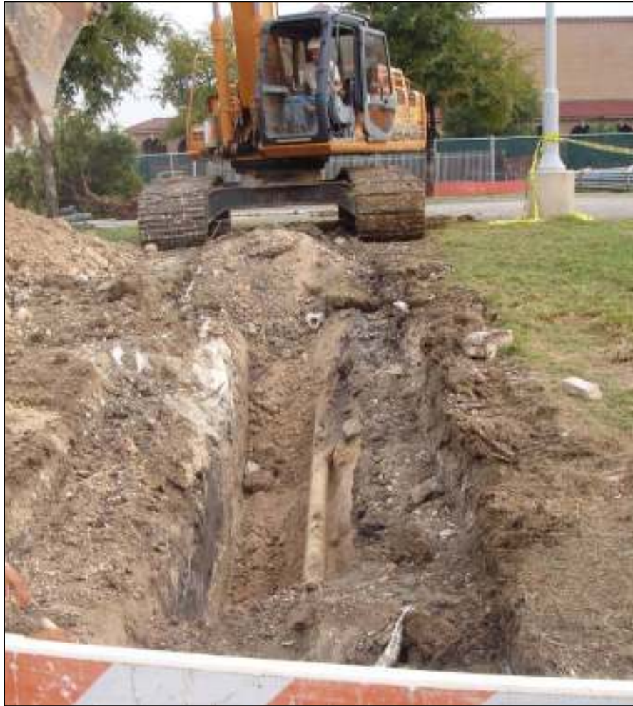
Figure 3-1. Photograph of mechanical excavation of utility trench, facing north.
