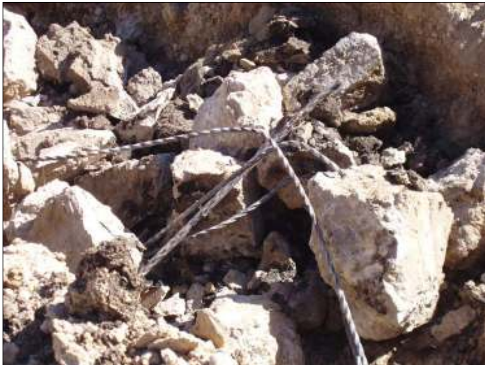
Figure 4-7. Photograph of the reinforced cement base of Feature 2.
